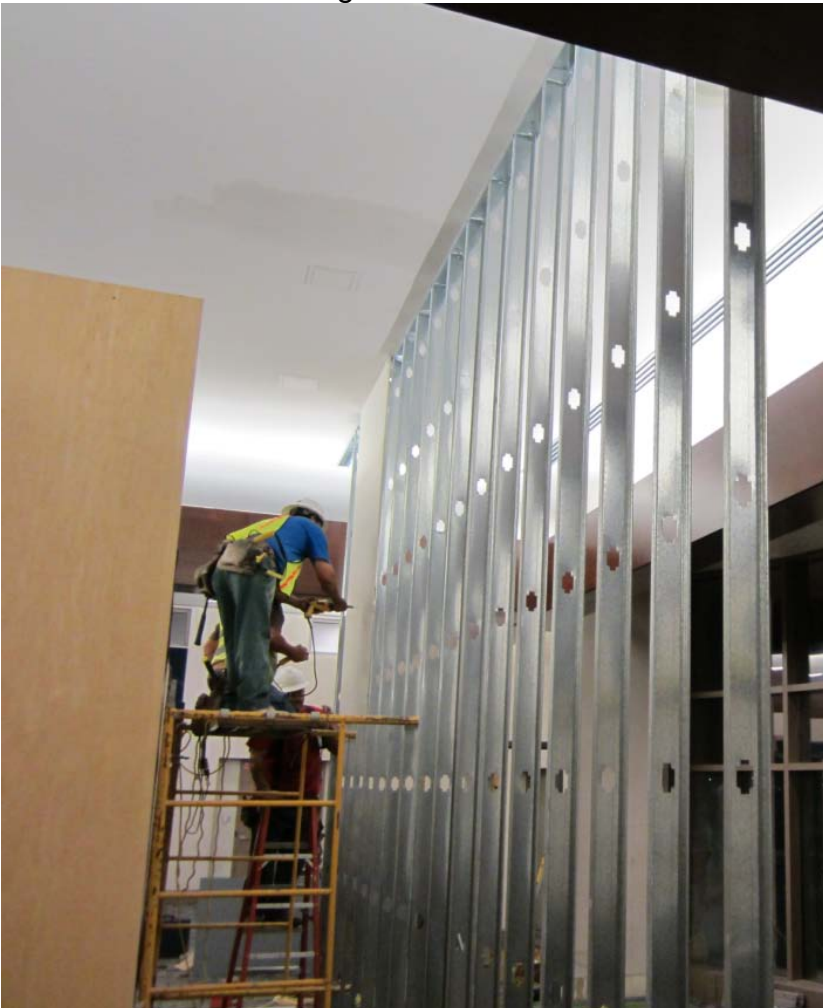
Construction of Demising Wall in Terminal Concourse
