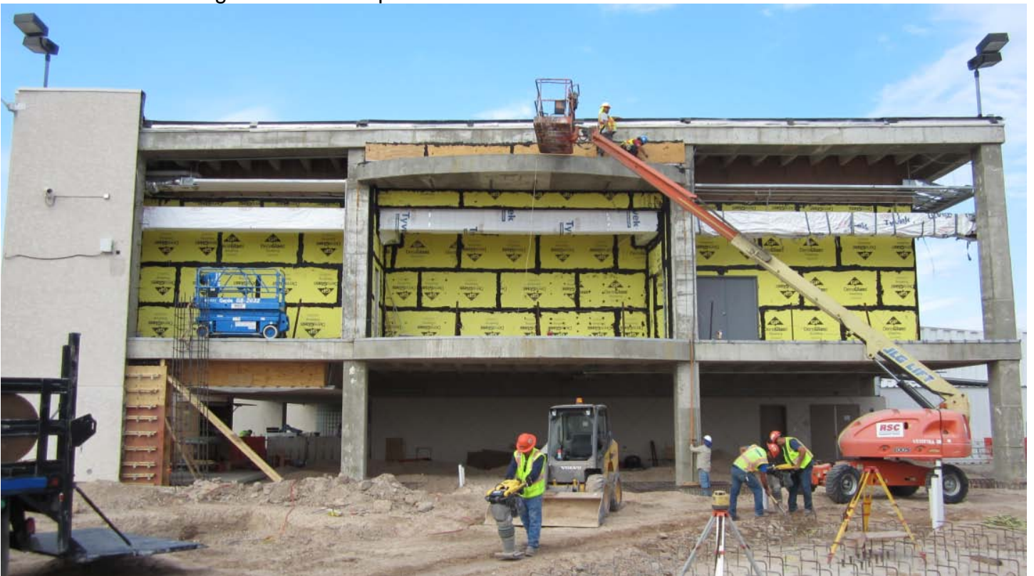
Terminal South Facing Removal Complete
