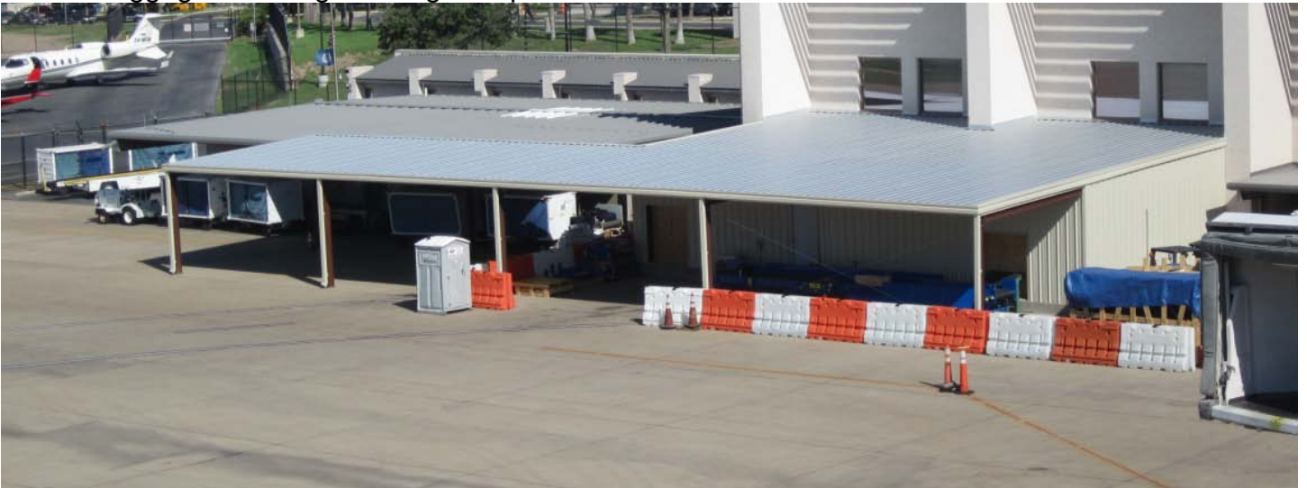
Interim Baggage Handling Building Complete
