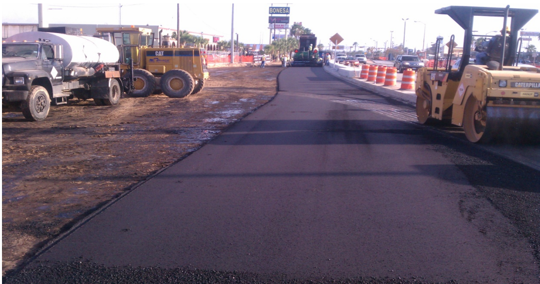
Placement of bond-breaker along Phase 2 looking northbound.
