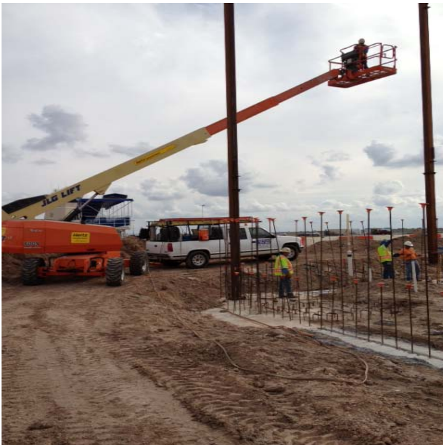
Steel erection – wall columns
