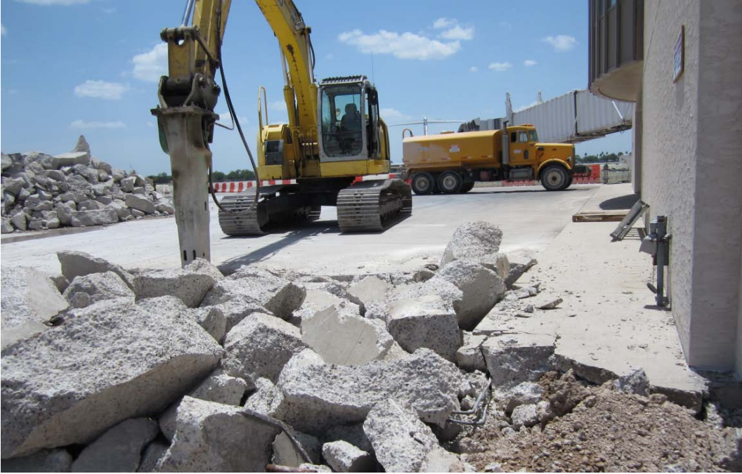
Demolition of Terminal Ramp
