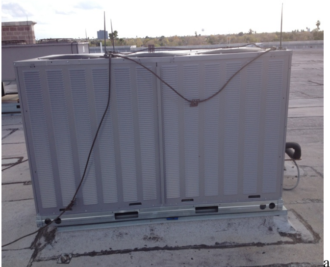
New Unit w/ Hail Guards (Public Safety Facility)
