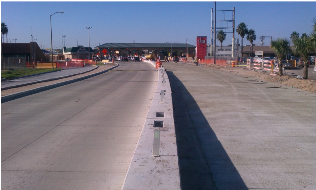
Concrete paving along Phase 2 looking southbound.
