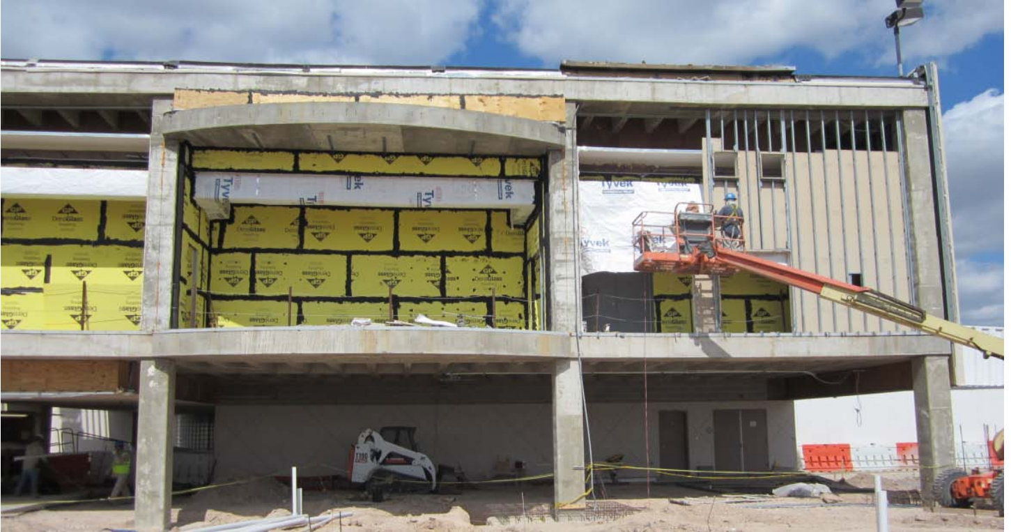
Terminal South Face Removal
