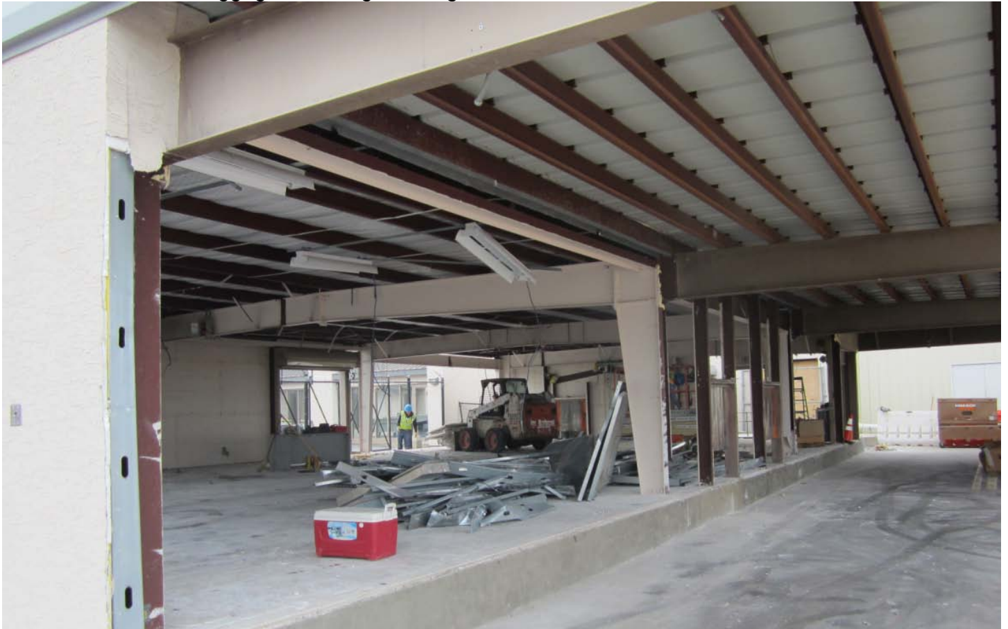
Demolition of "Old" Baggage Handling Building
