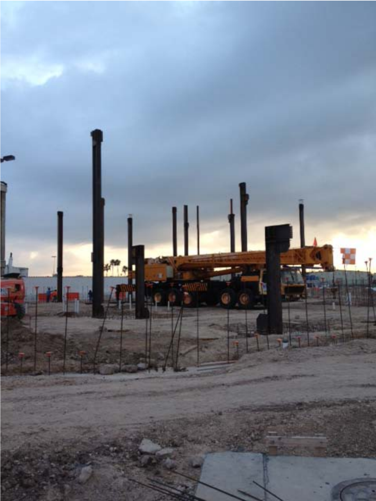
Terminal Steel Columns
