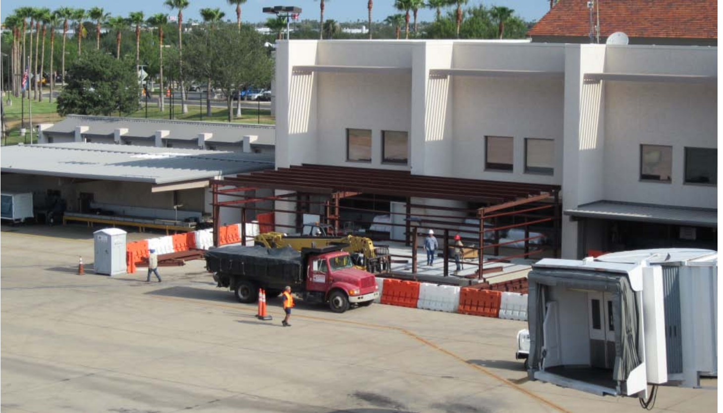
Interim Baggage Handling Building in Construction
