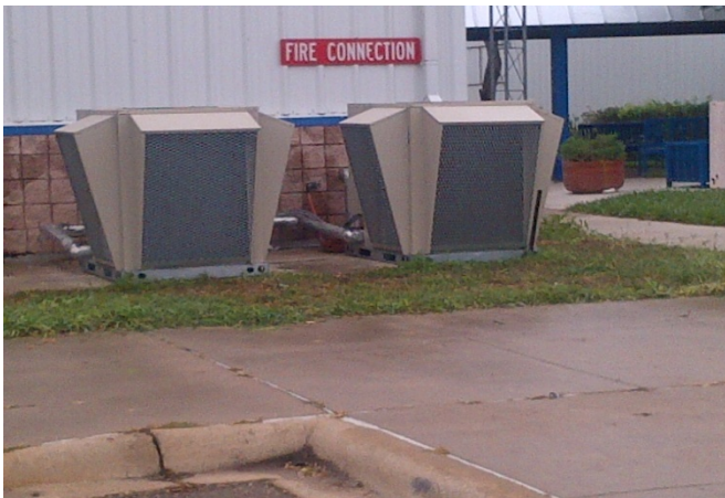
New Unit w/ Hail Guards (Public Works)
