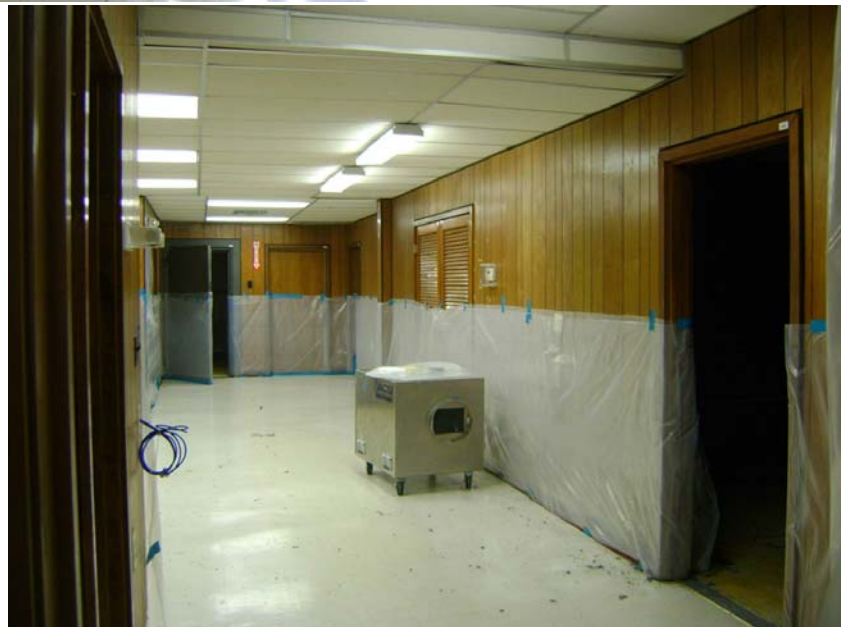
Typical sealing of corridor and air evacuation machine over tile to be removed.
