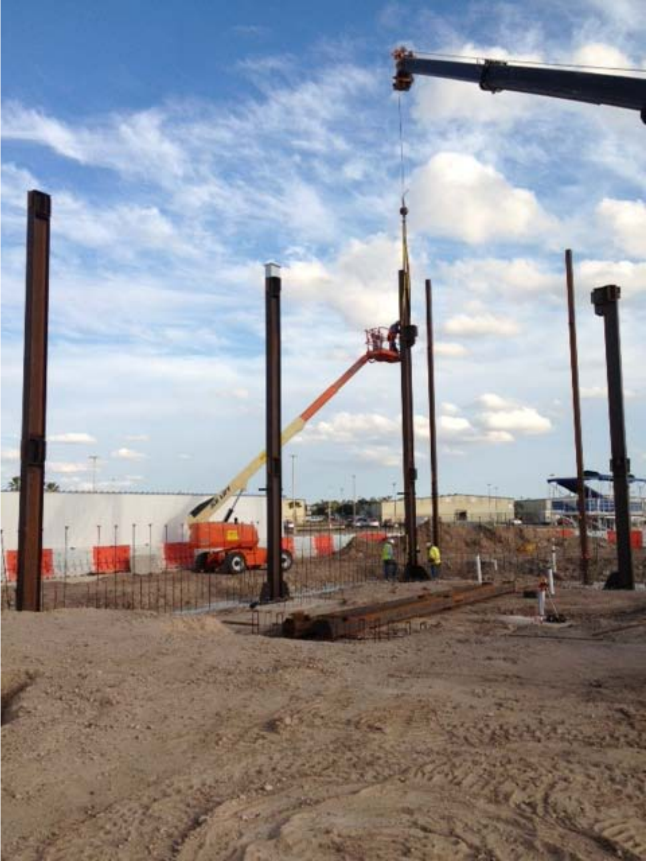
Steel erection – southern and eastern wall columns
