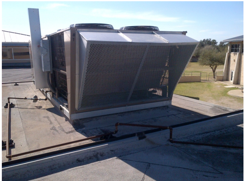
New Condenser Unit – Lark Community Center
