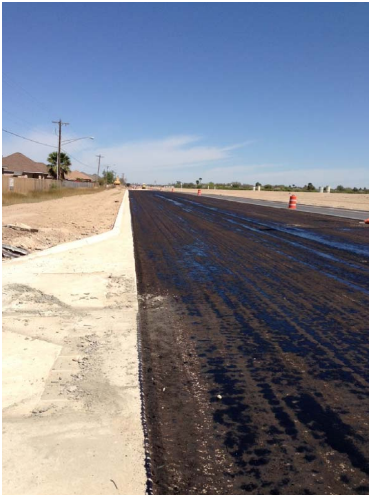
Flex-base is primed in preparation of laying asphalt from Pecan to Westway along the west side of Bentsen Rd (looking north).
