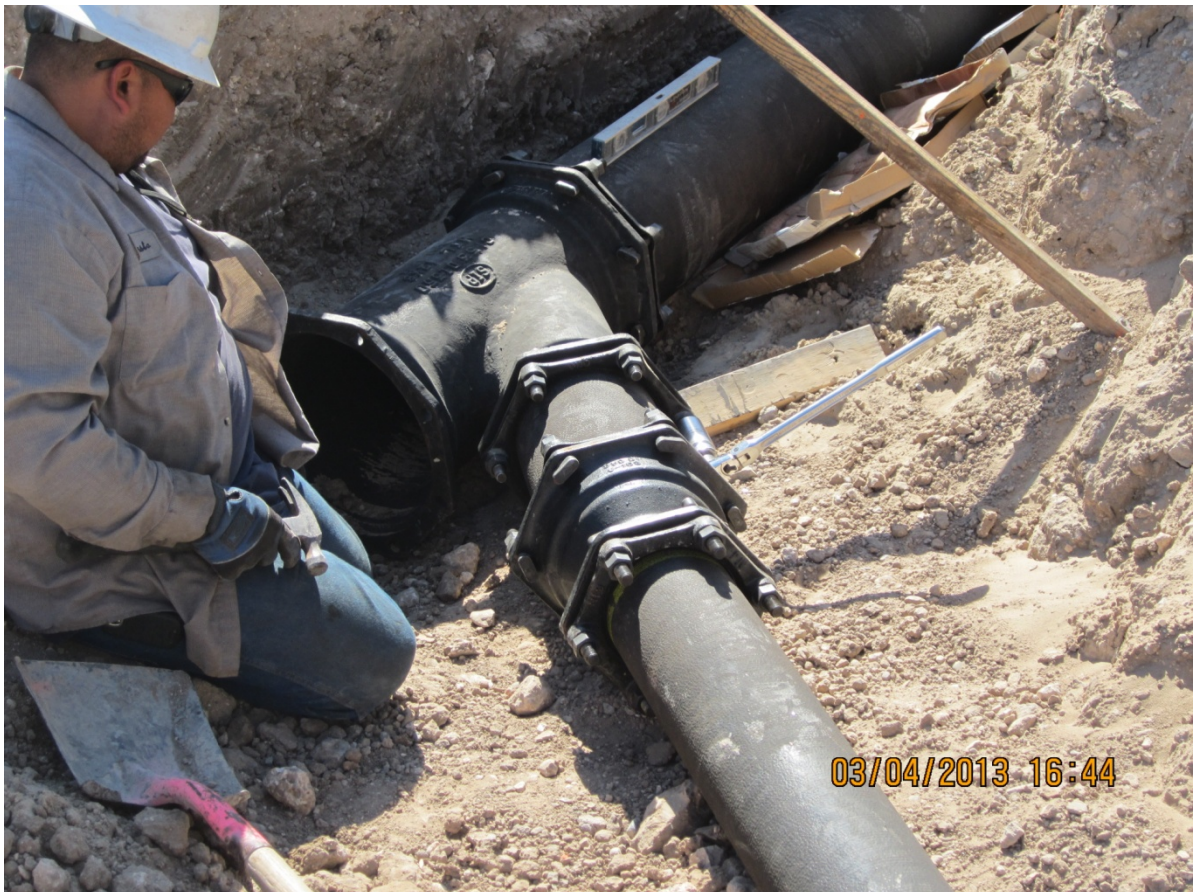
Installation of Storm Pipe for Roof Drains at Terminal Expansion
