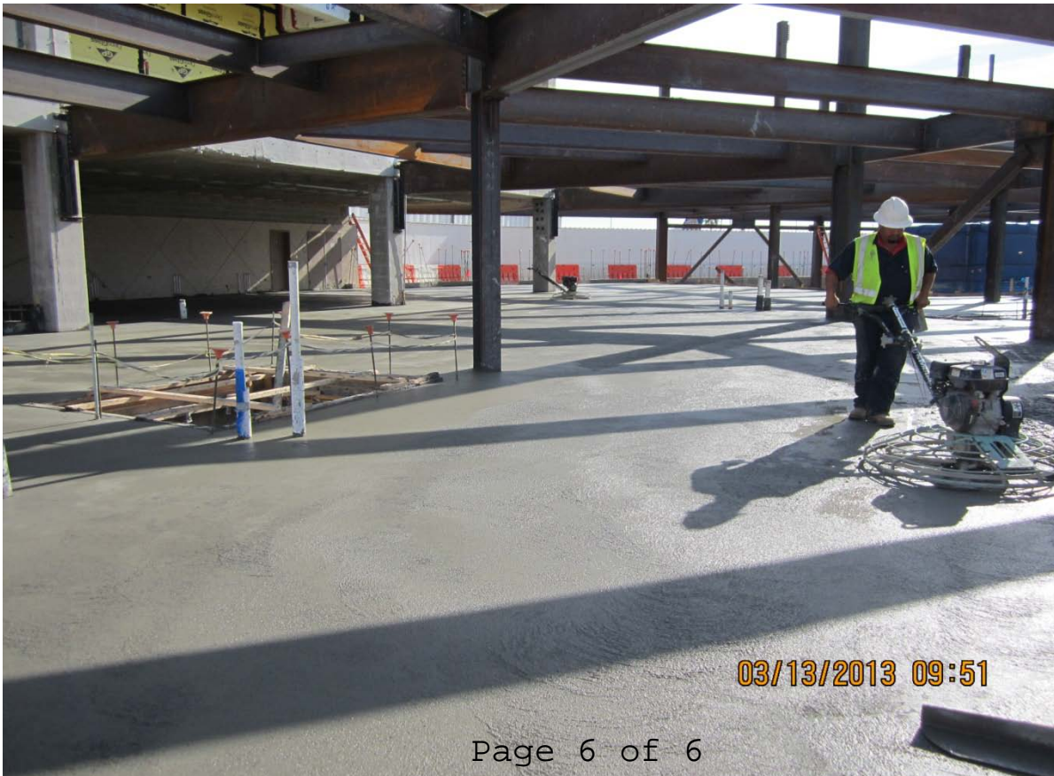
Concrete Finishing of First Floor Terminal Addition
