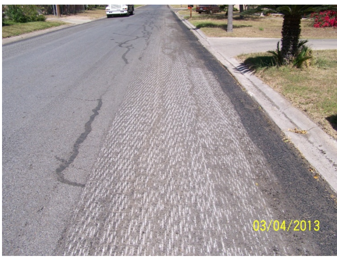
Typical view of street after curb milling and prior to repaving operations.
