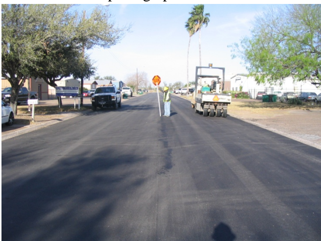
Typical view of completed street.
