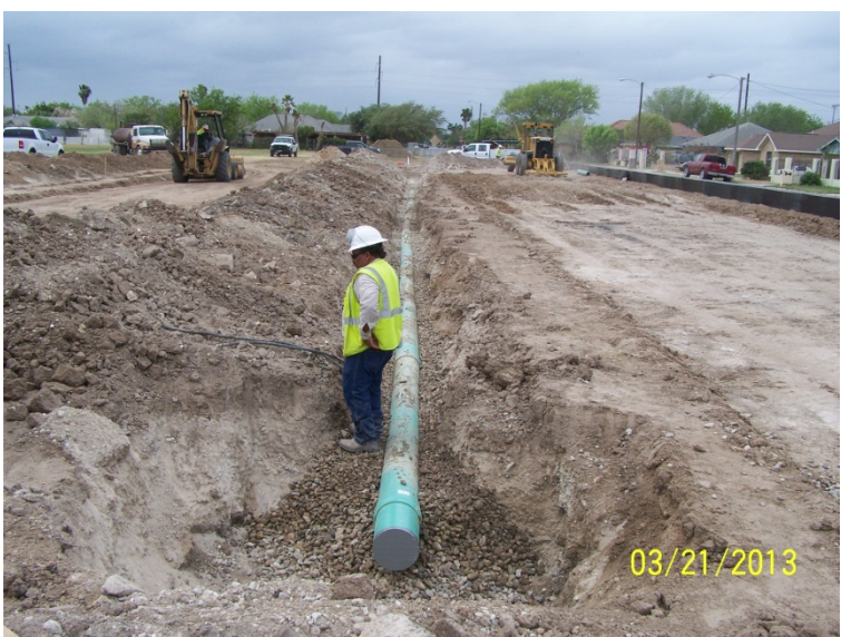
Storm Sewer Installation: Viewing West
