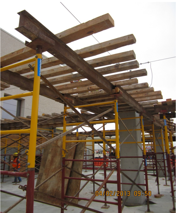
Formwork for the Second Story of the Permanent Baggage Handling Building
