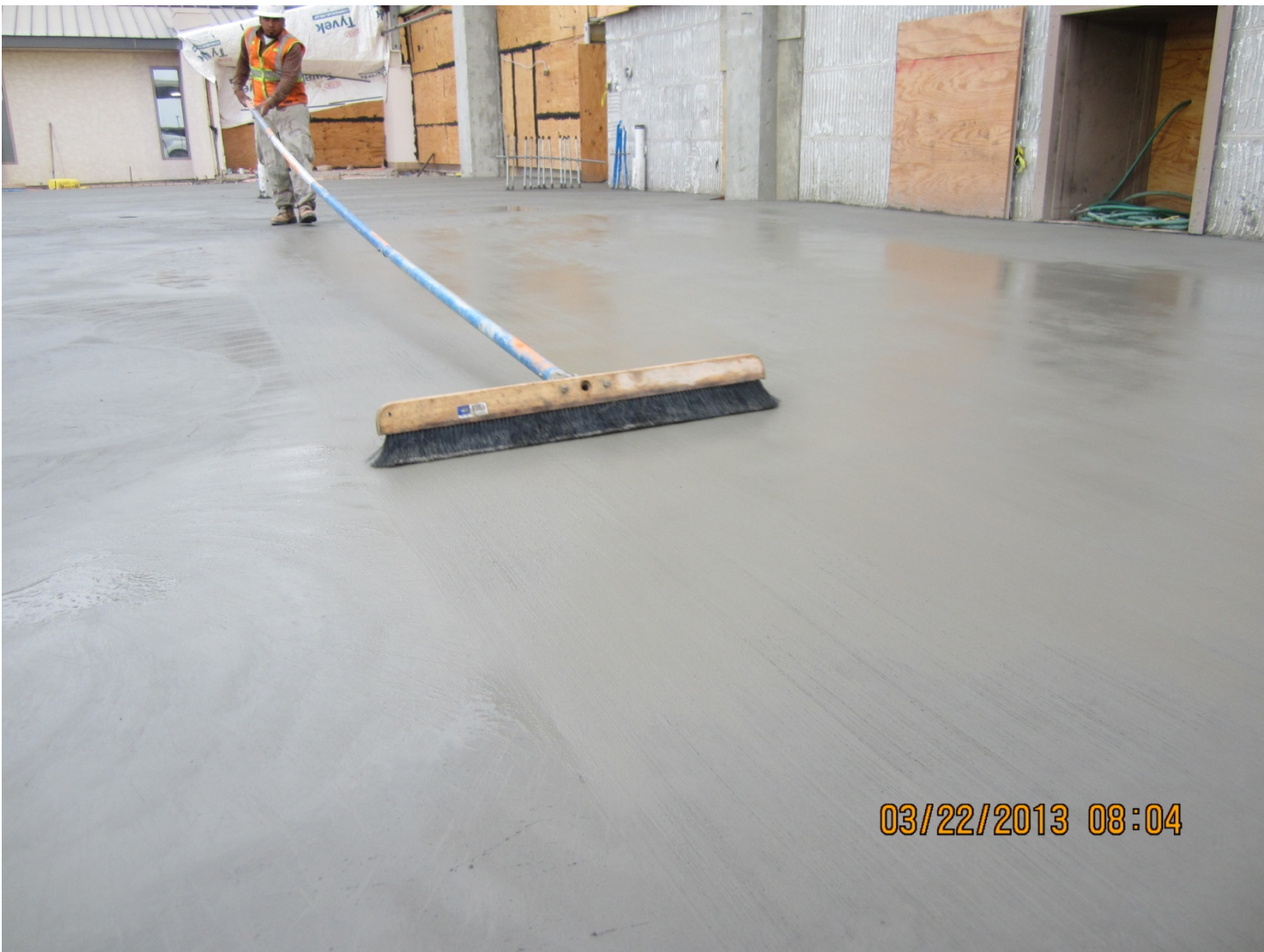
Concrete Finishing of First Floor at Permanent Baggage Handling Building
