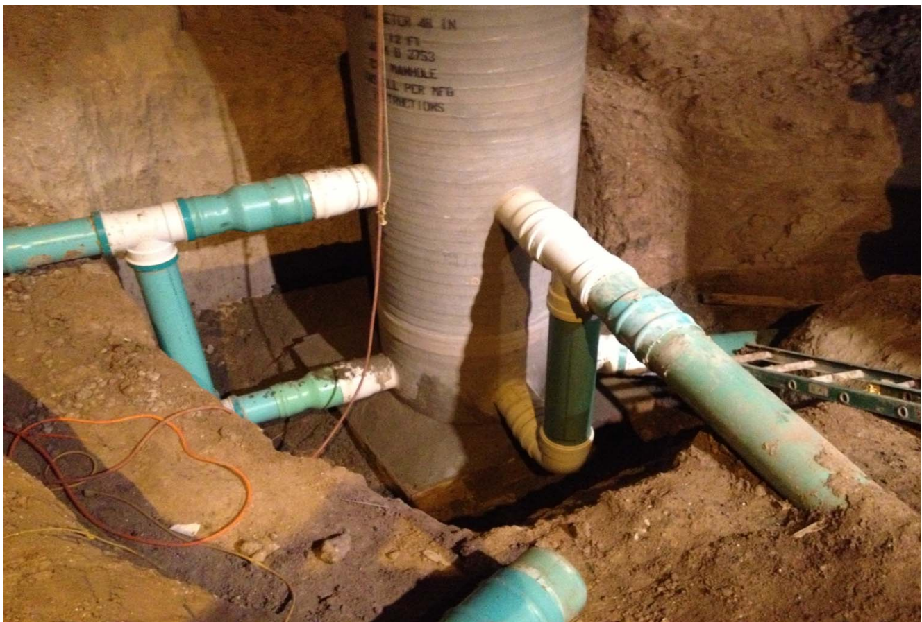
New sanitary sewer manhole with drop connections for serving adjacent subdivisions at Daffodil and 45 th Street.
