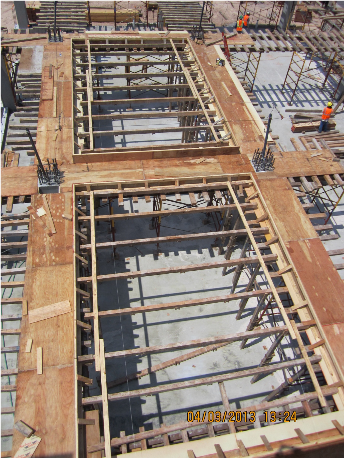
Top View of Formwork for the Second Story of the Permanent Baggage Handling Building
