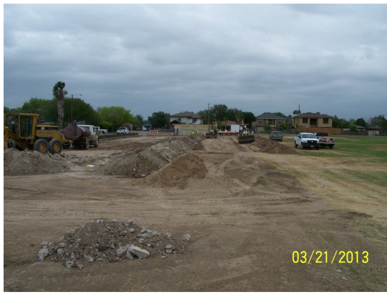
Site Clearing and Preparation: Viewing East
