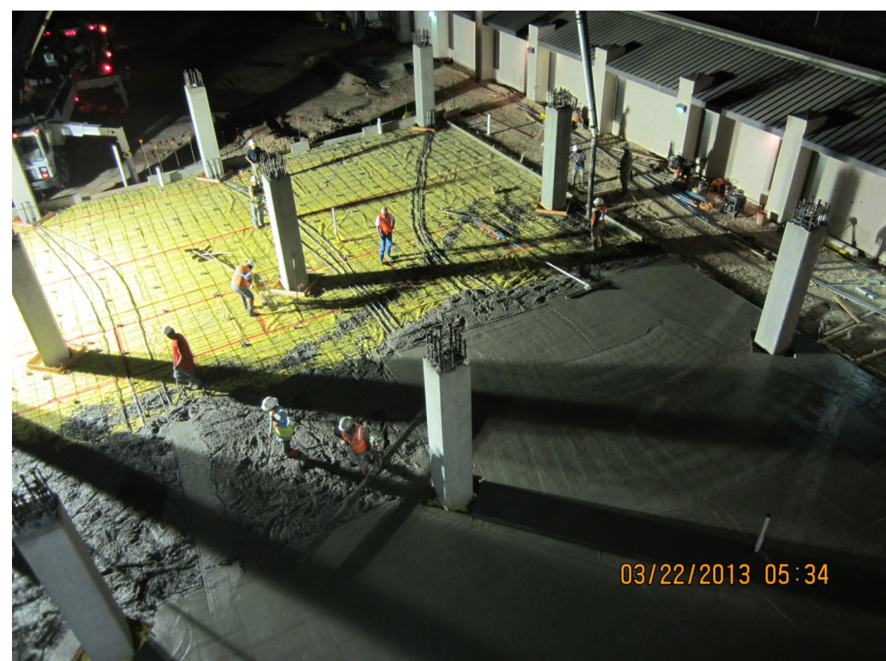
Concrete Pour on First Floor at Permanent Baggage Handling Building
