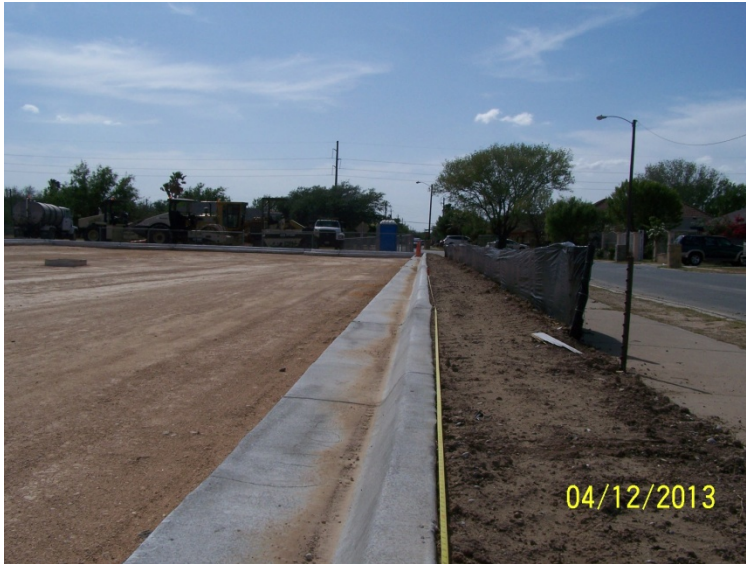
North Parking Lot Curb Line: Viewing West
