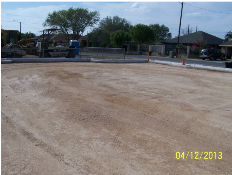
Completed Base: Viewing Northwest
