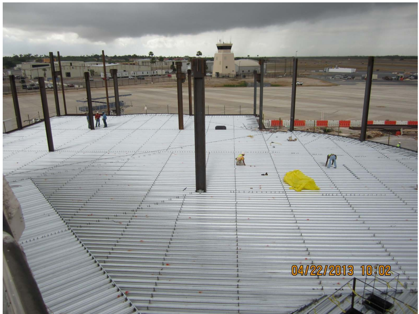
Completed metal decking on second story of Terminal Expansion
