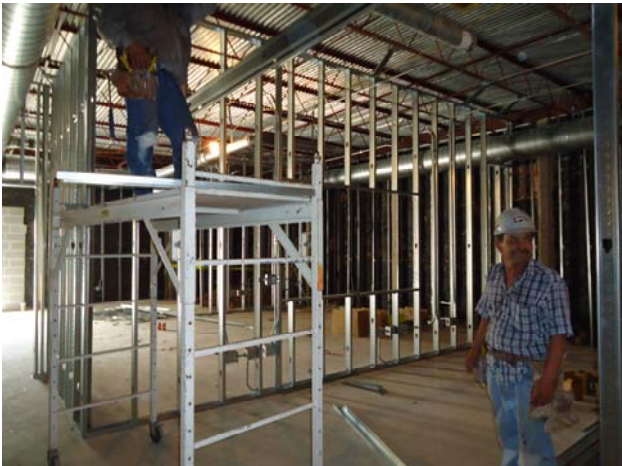
Interior alum. Stud wall, duct placement
