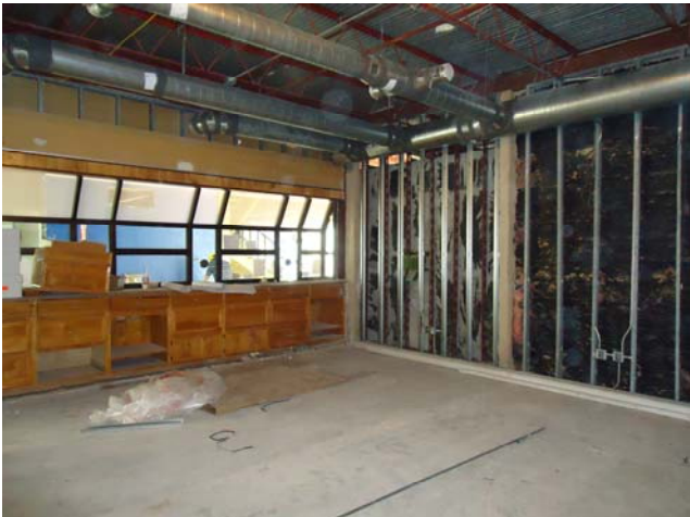
Interior of tax office
