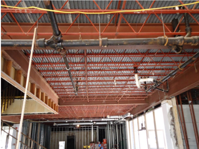
Exposed structural elements – central pod
