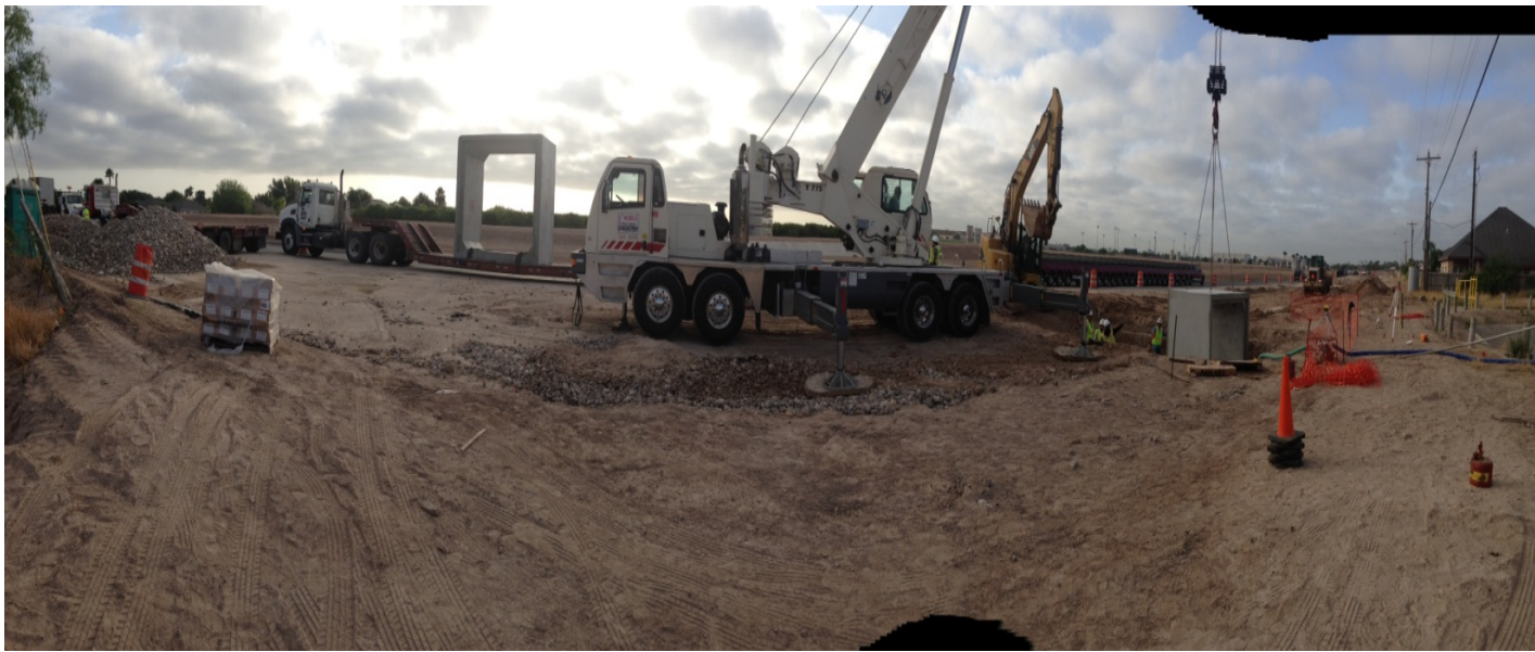
Installation of 10' X 10' Reinforced Concrete Boxes as part of 2012 Hidalgo County Drainage Bond.
