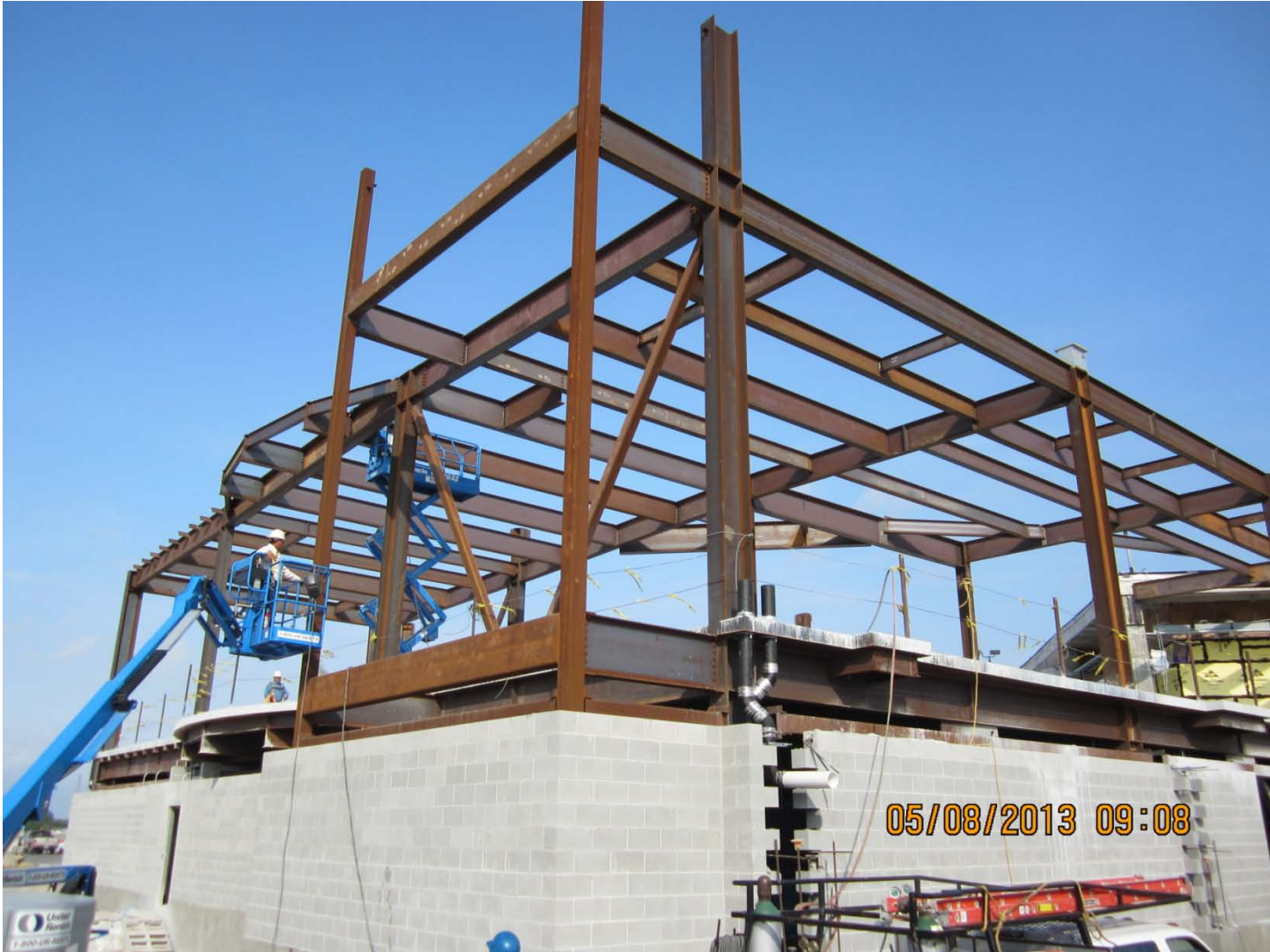
Roof steel erection at Terminal Expansion
