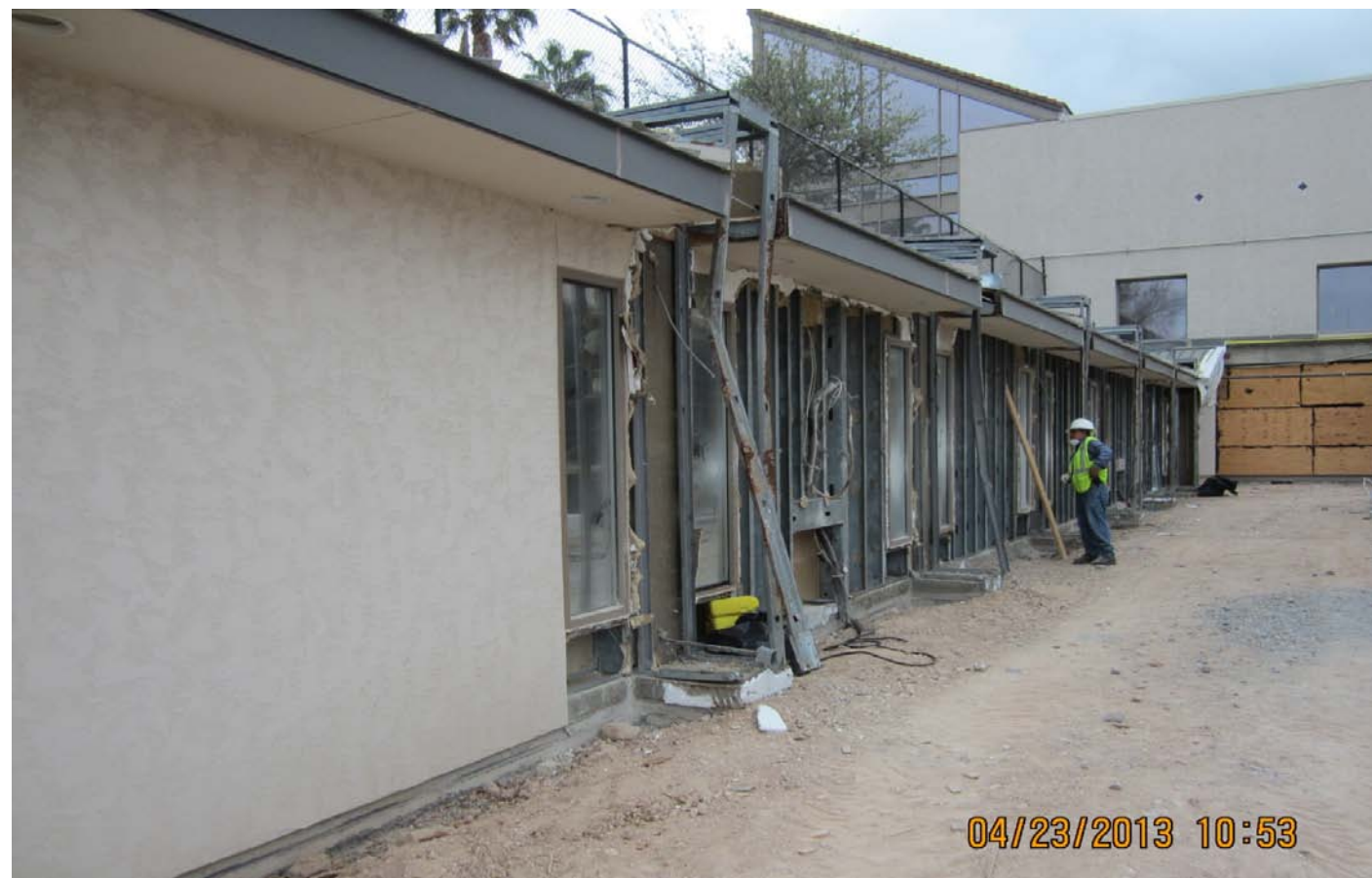
Demolition of Federal Inspection Walkway at the Baggage Handling Building
