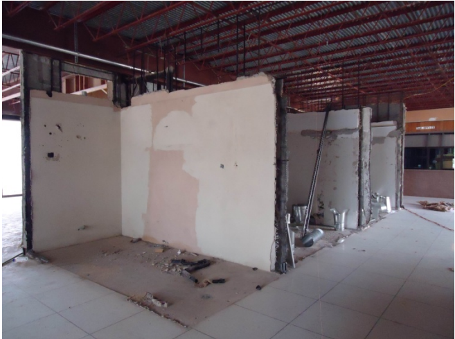
Plaster walls to be demolished
