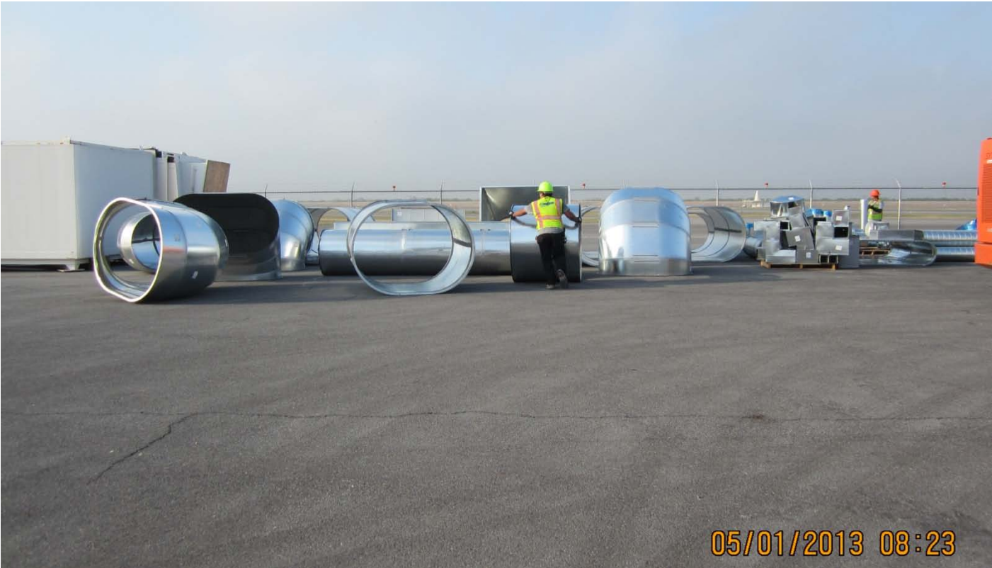
Delivery of HVAC duct work for installation in Terminal Expansion
