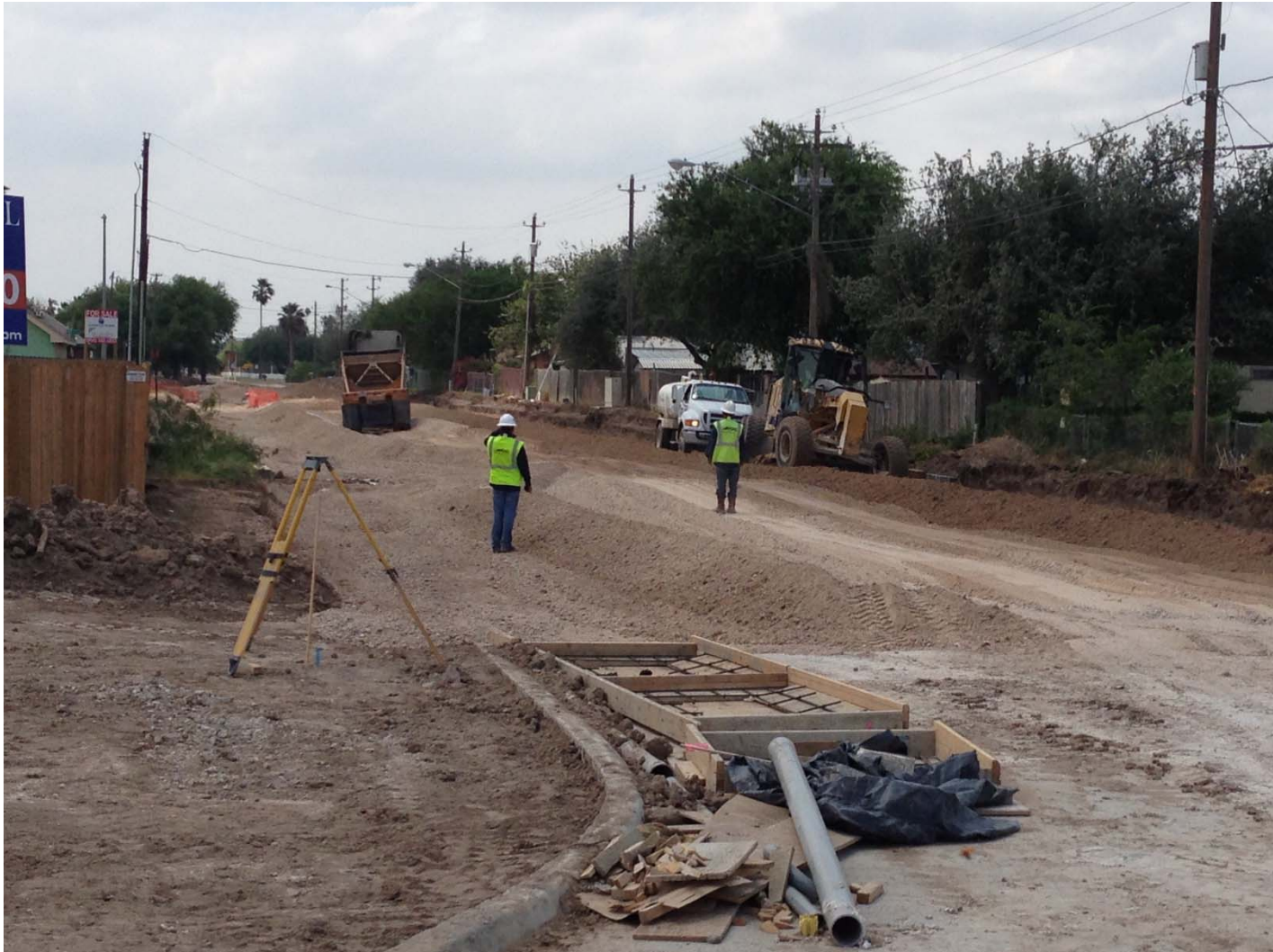
Installation of 10' X 10' Reinforced Concrete Boxes as part of 2012 Hidalgo County Drainage Bond.
