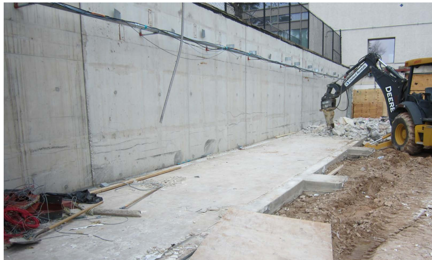
Foundation demolition of Federal Inspection Walkway at the Baggage Handling Building
