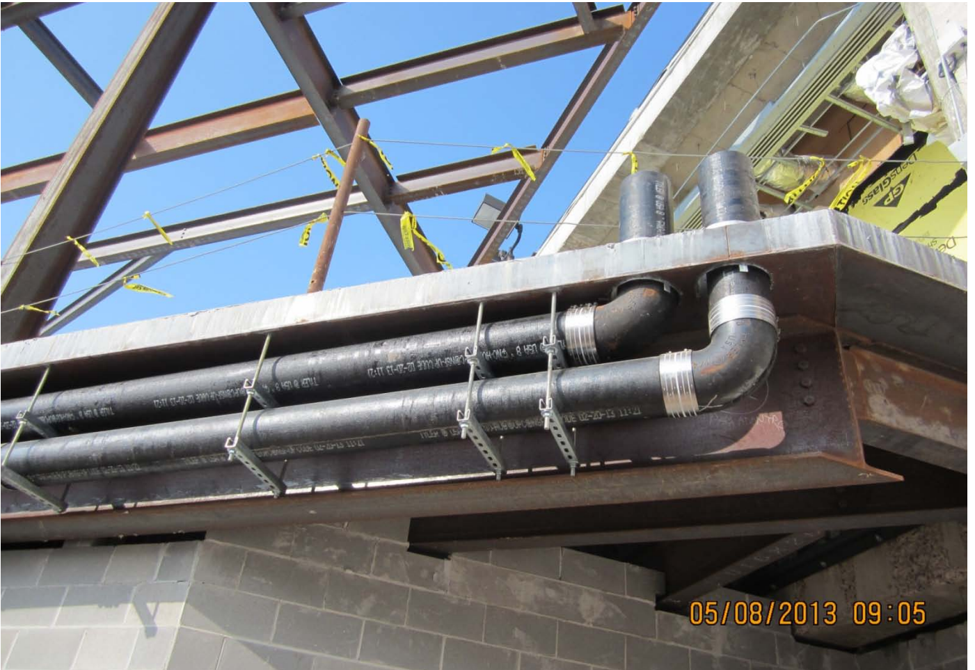
Roof Drains for Terminal Expansion
