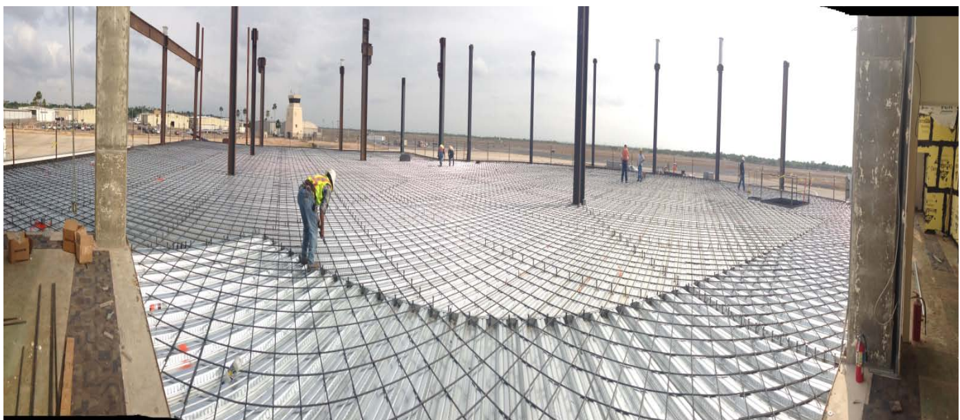
Installation of steel reinforcement mat over metal decking on second story of Terminal Expansion
