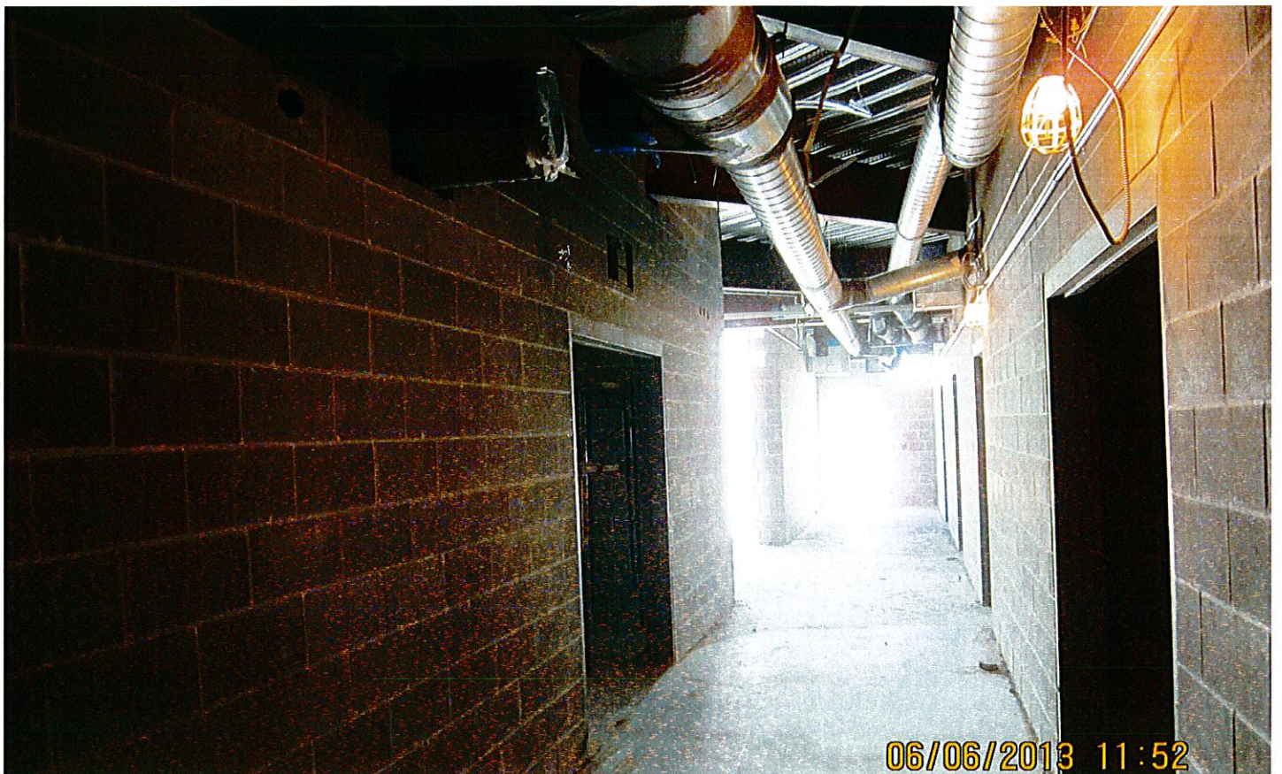
Ductwork within hallways on First Floor of Terminal Expansion
