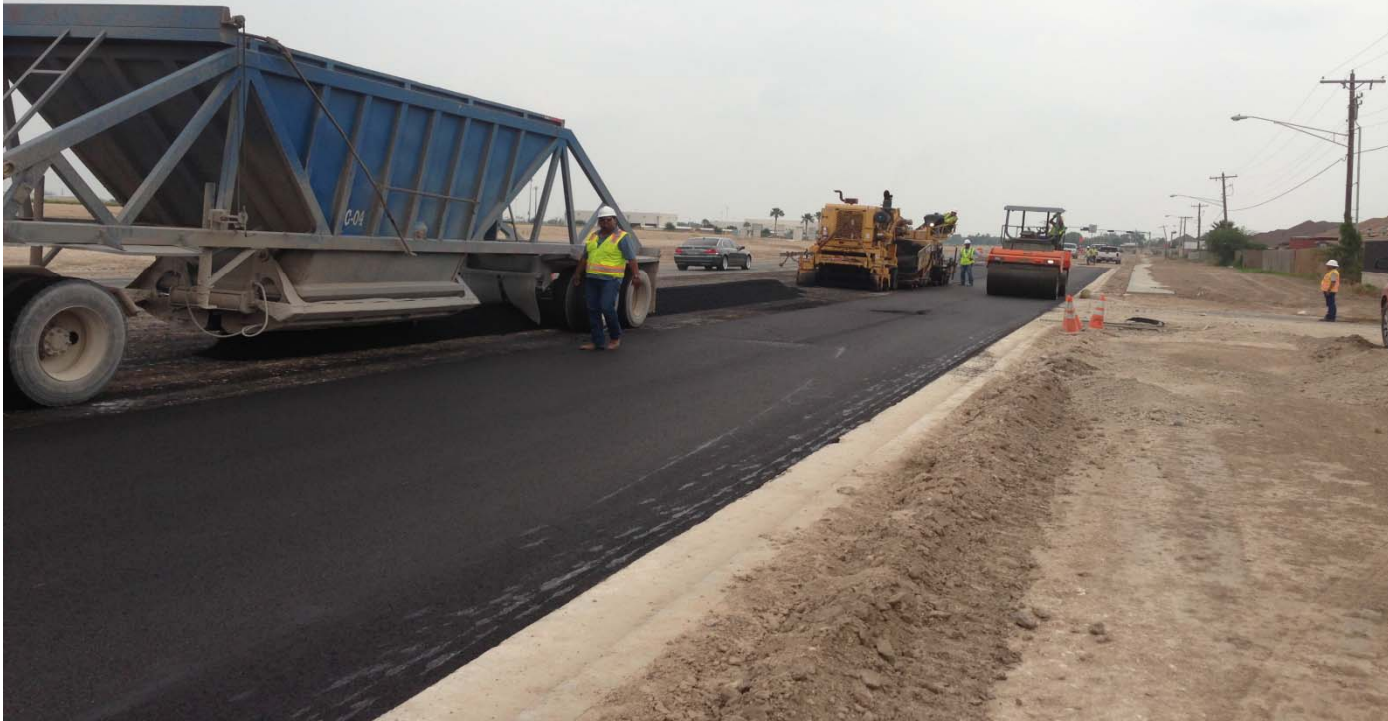
Paving operations of the west side of Bentsen Road from Vine to Nolana.
