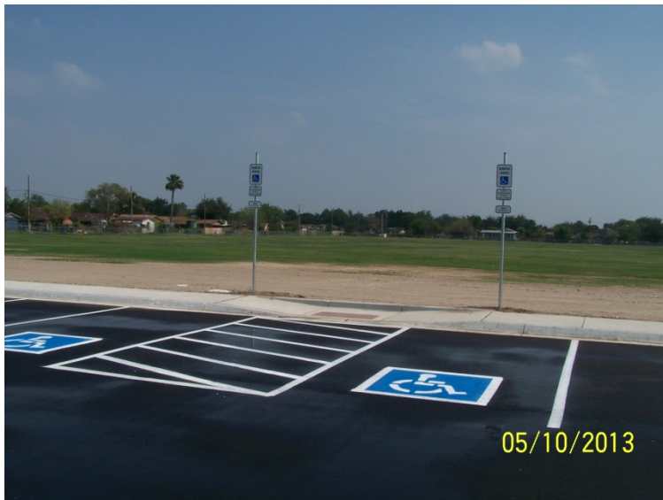
South Parking Lot Curb Line: Viewing South
