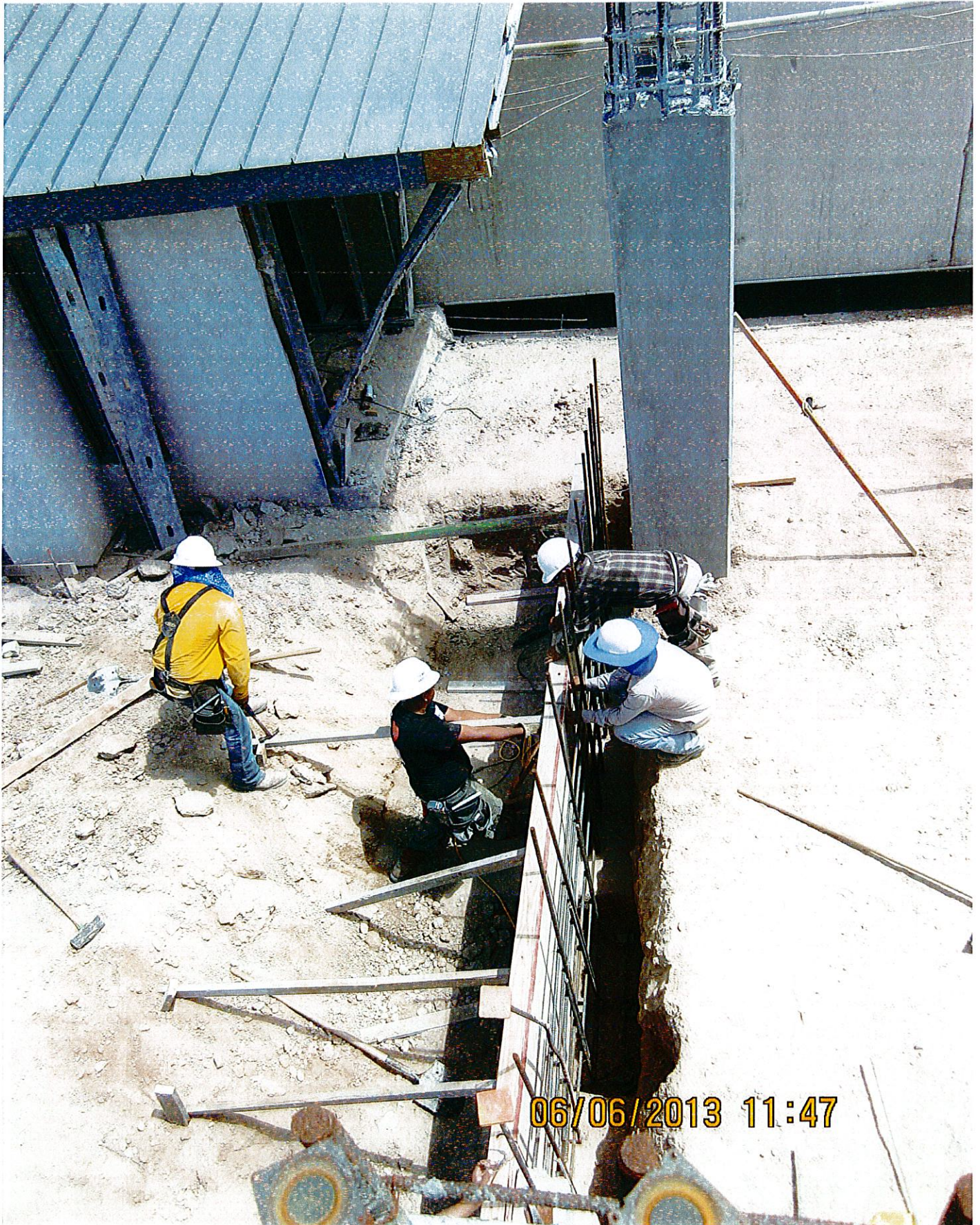
Forming and steel reinforcement placements in preparation of remainder of foundation pour at Baggage Handling Building
