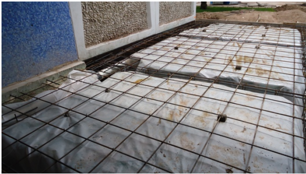
Eastern foundation pad – pre-pour
