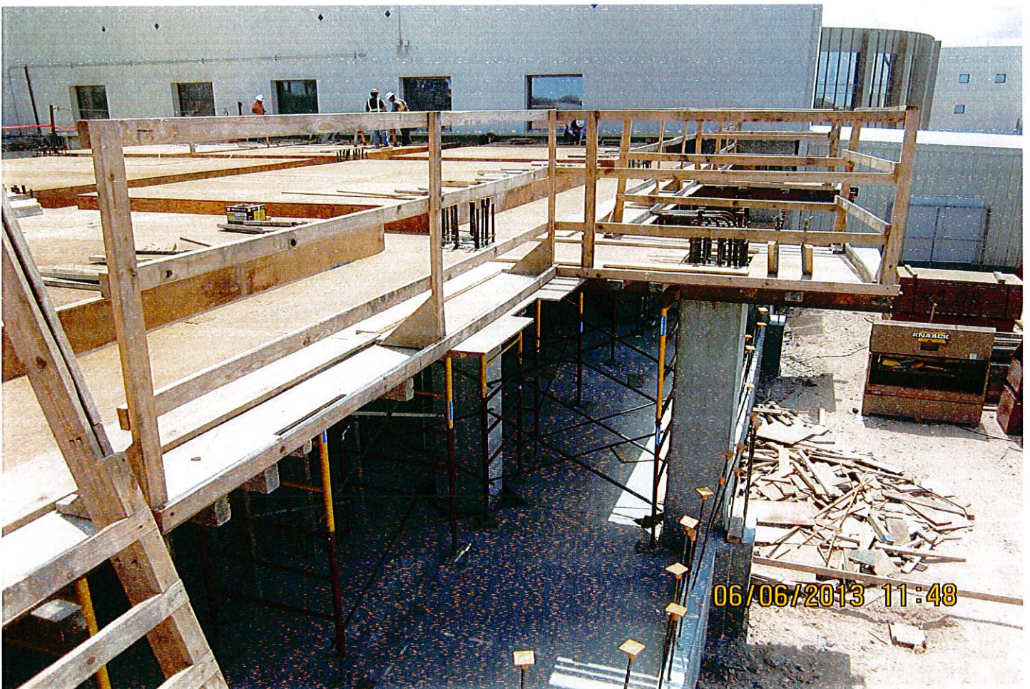
Forming and steel reinforcement placements in preparation of elevated slab at Baggage Handling Building
