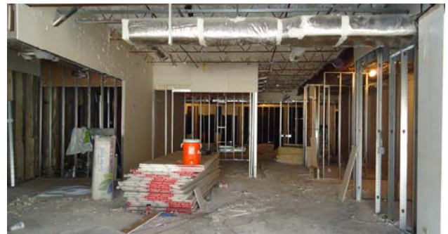
Level of progress in pod
