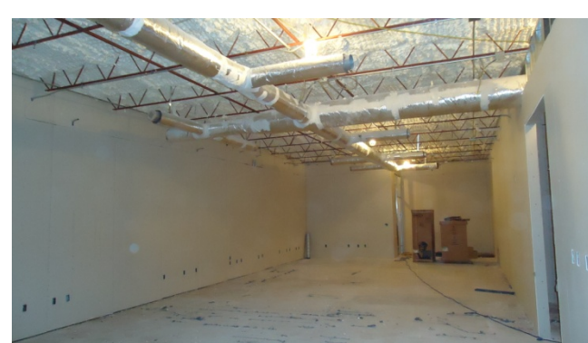
Interior progress – below deck insulation, gypsum board application, AC ducts, electrical conduit and wiring
