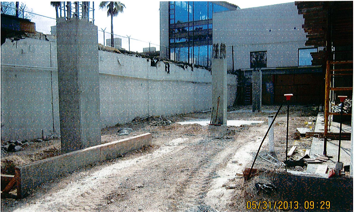
Completion of footings and columns at the Baggage Handling Building
