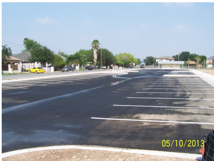
Completed Parking Area: Viewing East
