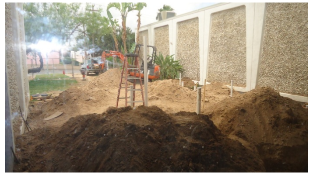
Southern foundation pad - preparation
