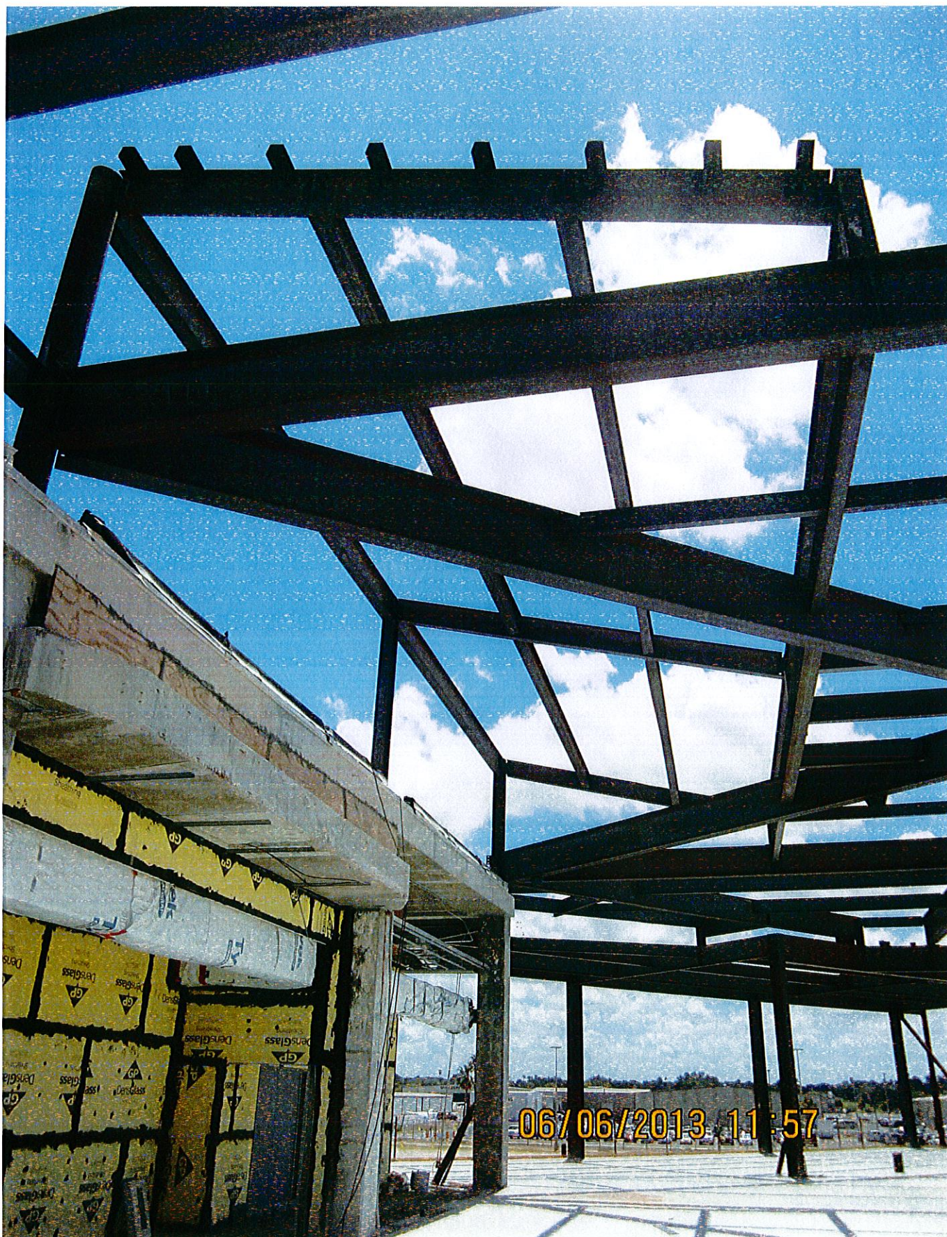
Structural steel for roof above Second Floor of Terminal Expansion
