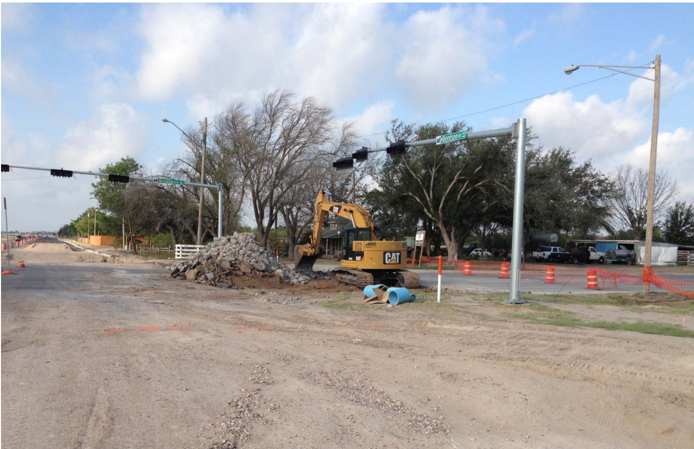
Preparation of the west leg at the intersection of Nolana and Bentsen looking southwest.
