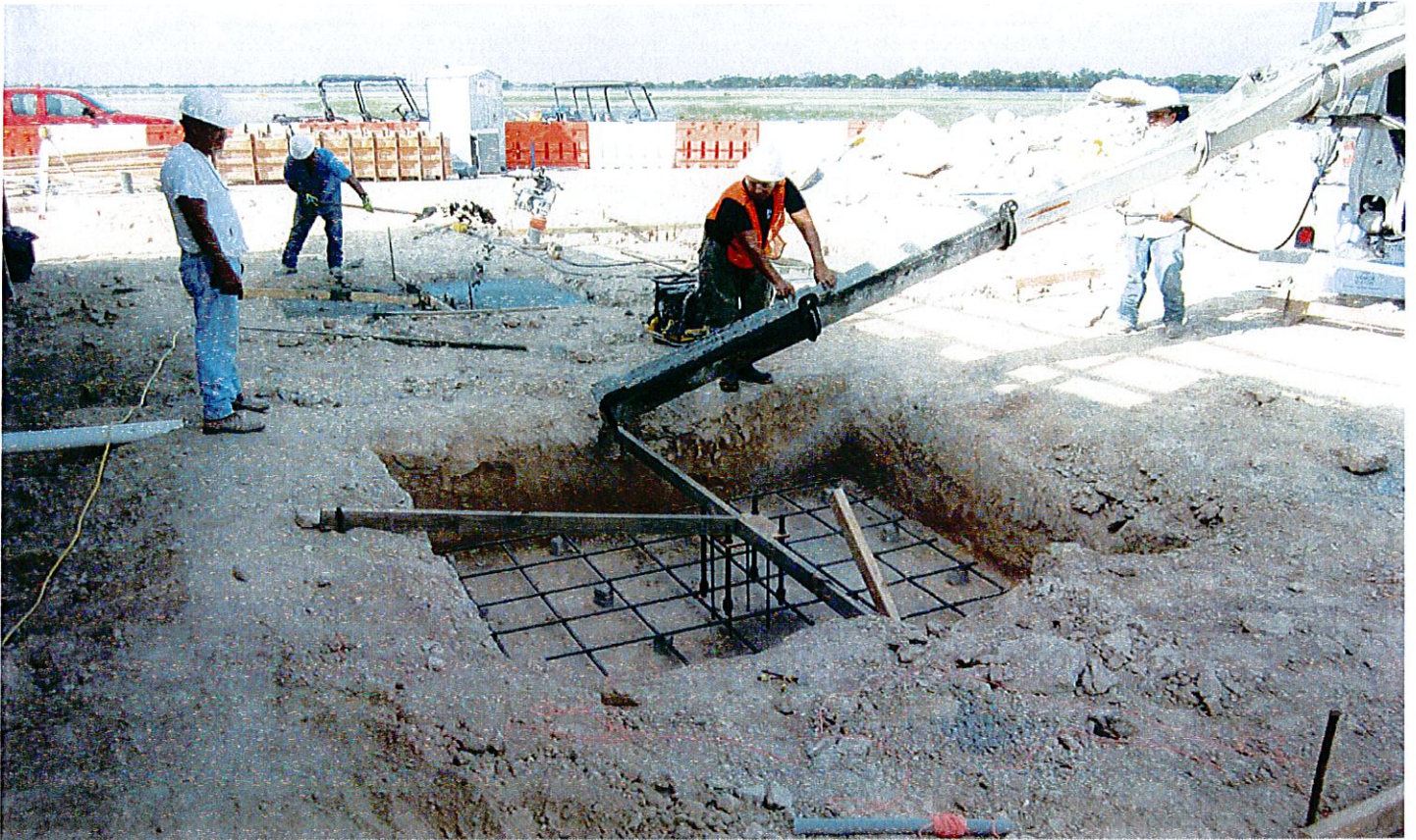
Pouring concrete for structural footings at the Baggage Handling Building
