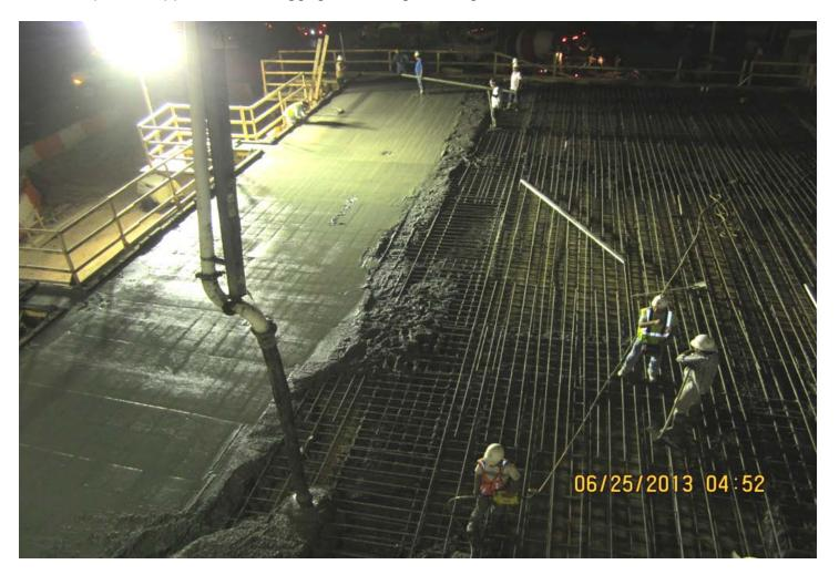
Concrete finishers as completion of pour at upper level of Baggage Handling Building nears
