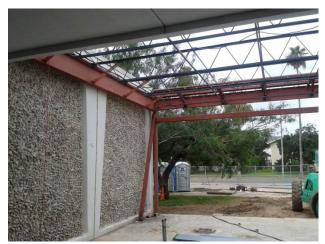
Eastern foundation pad and structural steel
