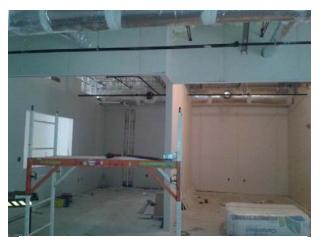
Interior progress – below deck insulation, gypsum board application, AC ducts, electrical conduit and wiring, fire sprinkler
