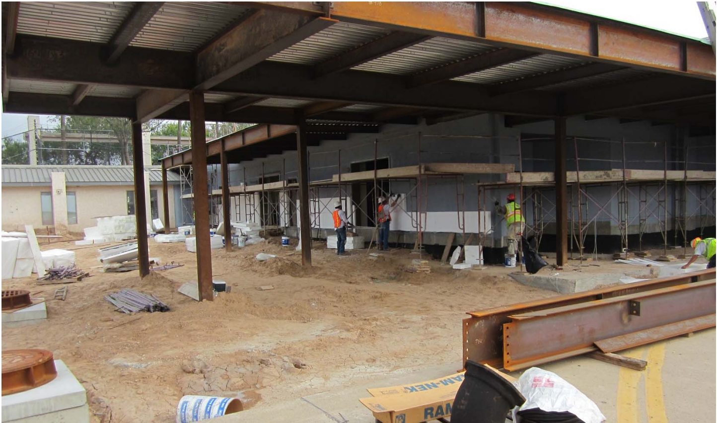
Insulation preparation for exterior EIFS at the Baggage Handling Building
