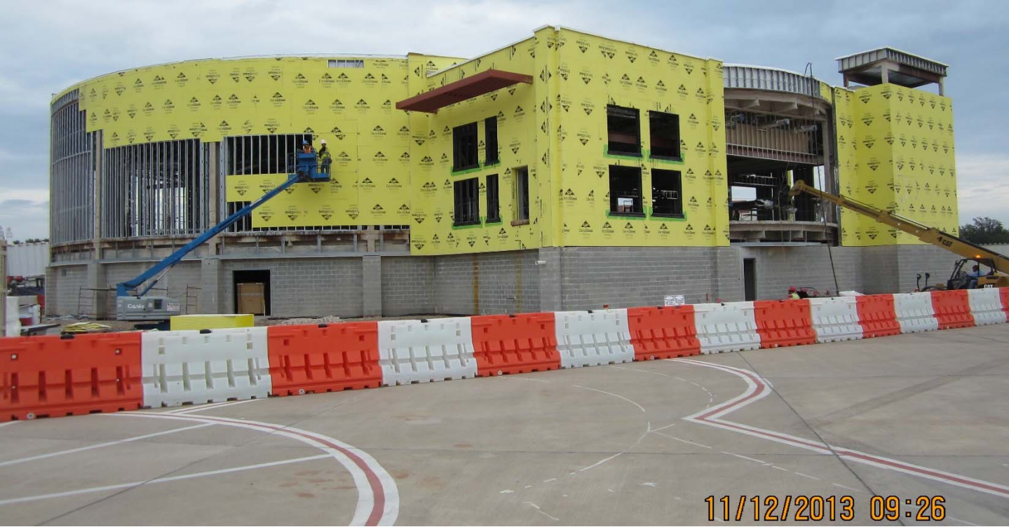
Installation of sheathing of exterior on south end of Terminal Expansion
