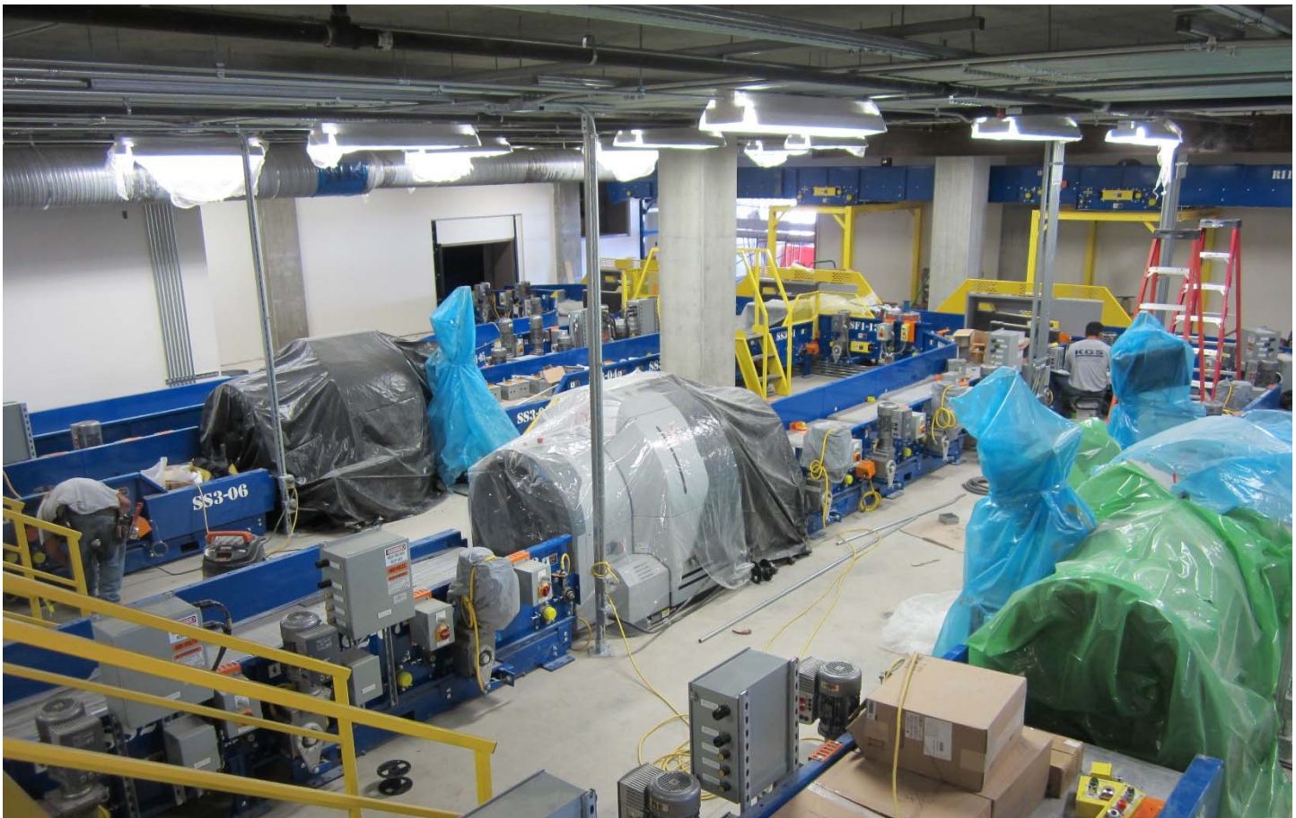
Conveyor lines with new TSA security equipment at Baggage Handling Building
