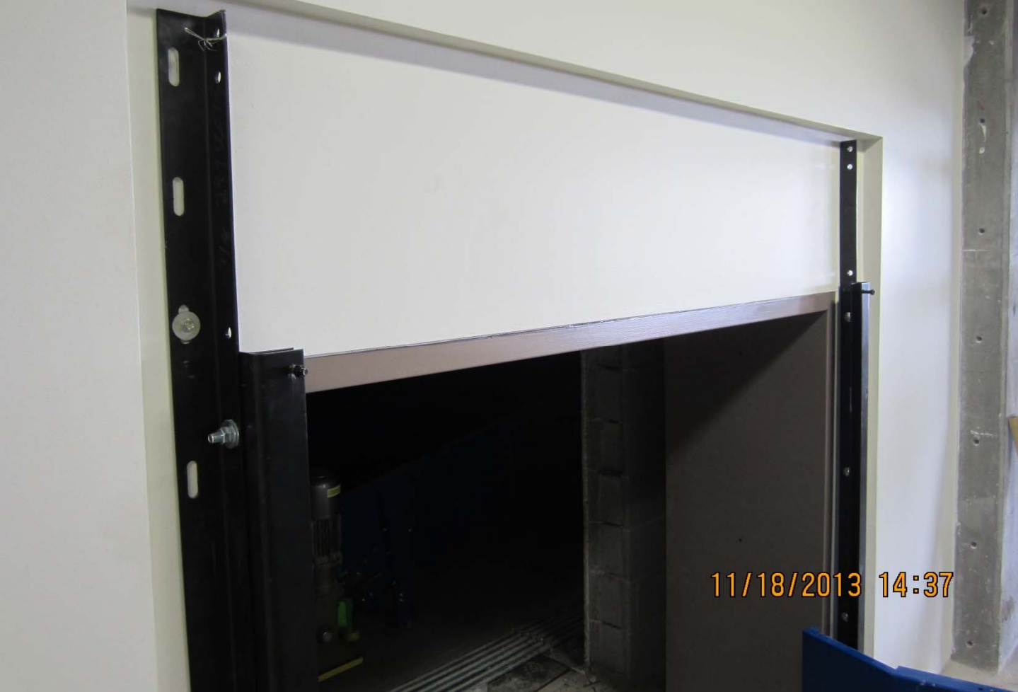
Conveyor wall opening at the Baggage Handling Building
