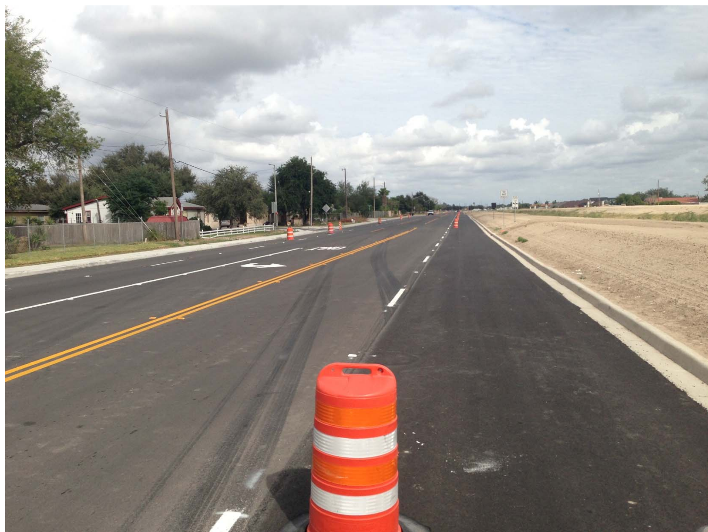
Paving with final striping complete looking northbound from Daffodil.
