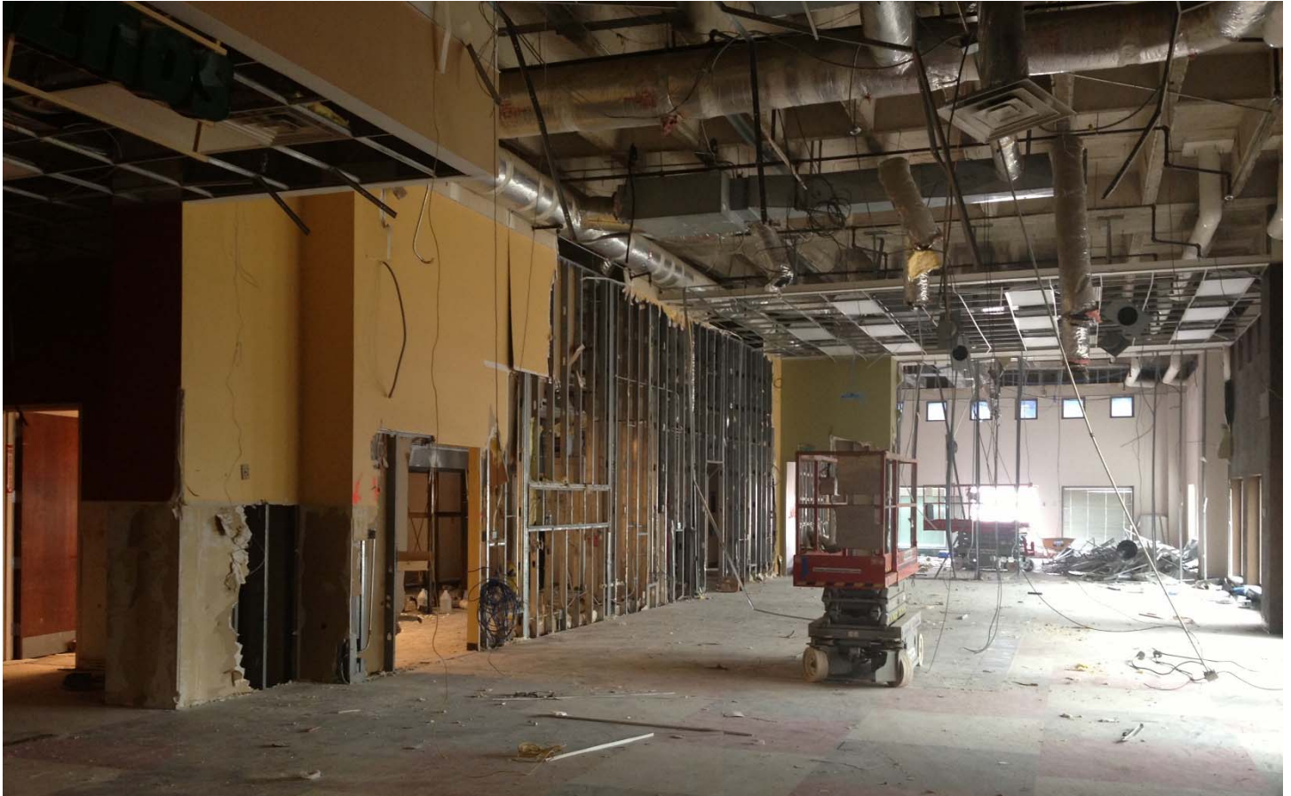
Demolition work for future TSA offices within the Terminal Expansion
