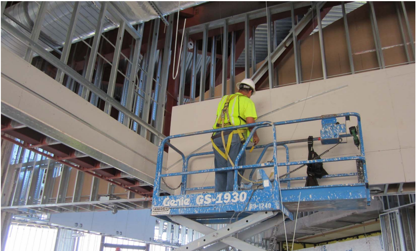
Interior wall construction at upper level of Terminal Expansion
