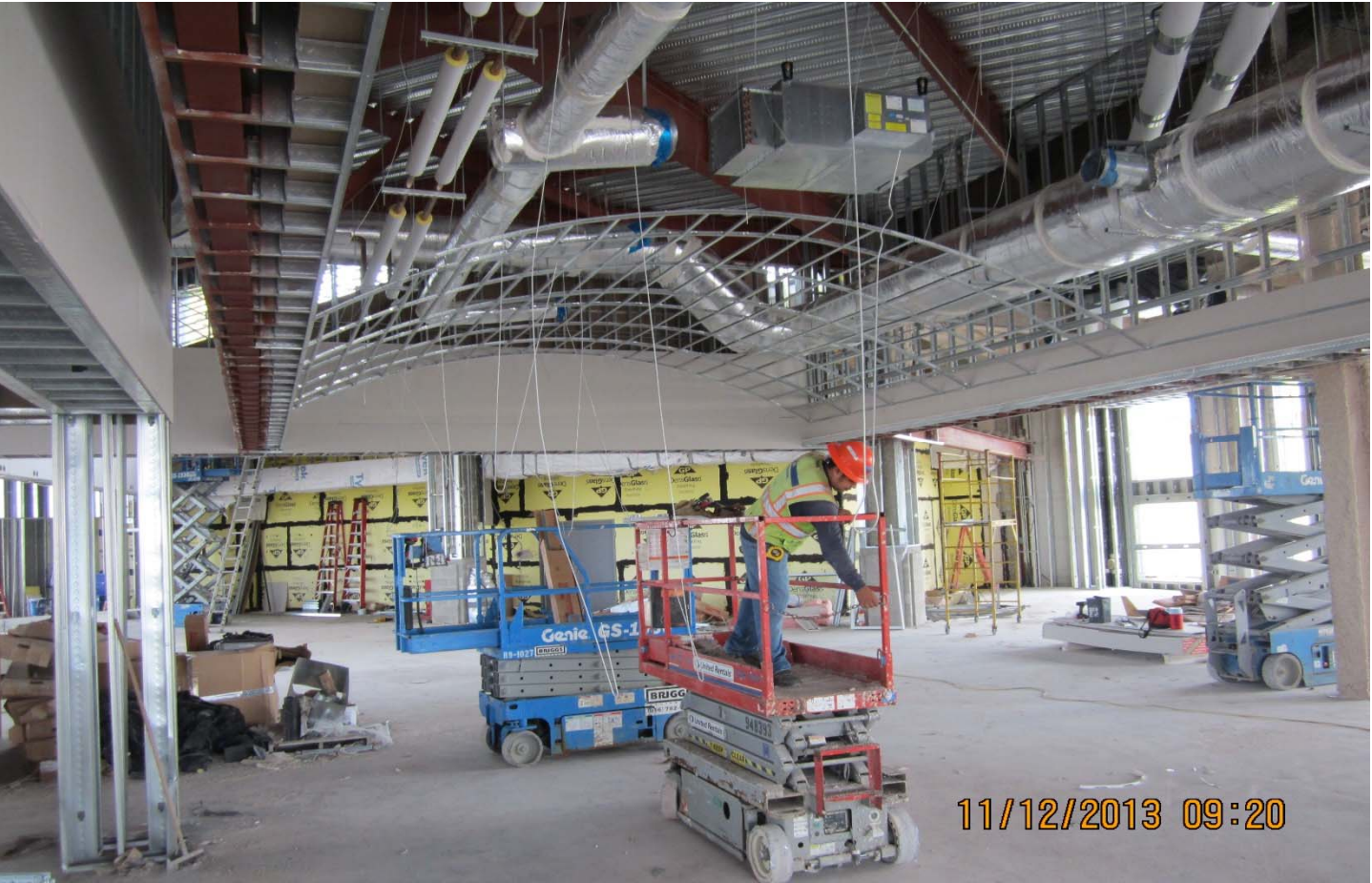
Installation of barrel ceiling at upper level Terminal Expansion
