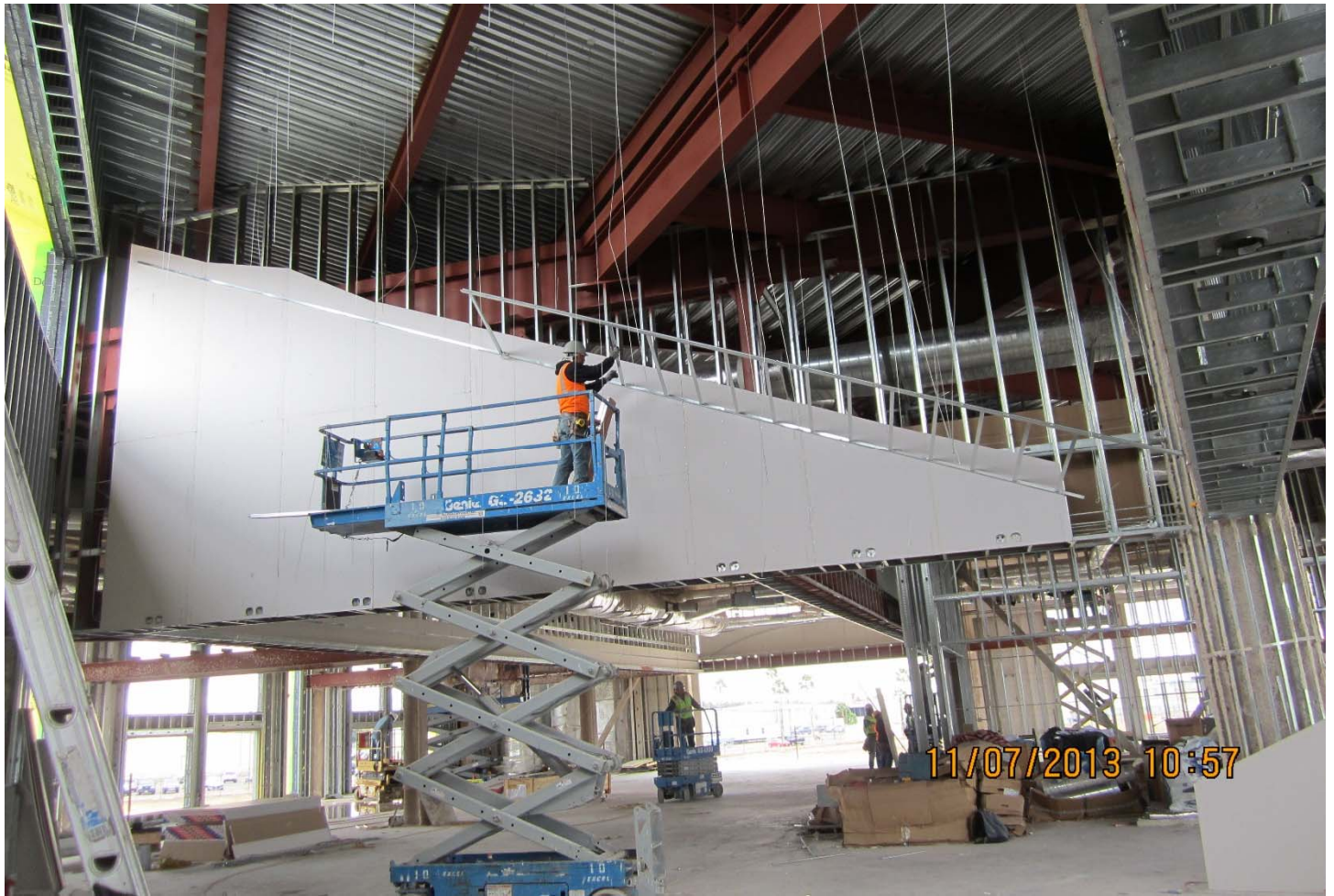
Installation of ceiling grid at upper level Terminal Expansion
