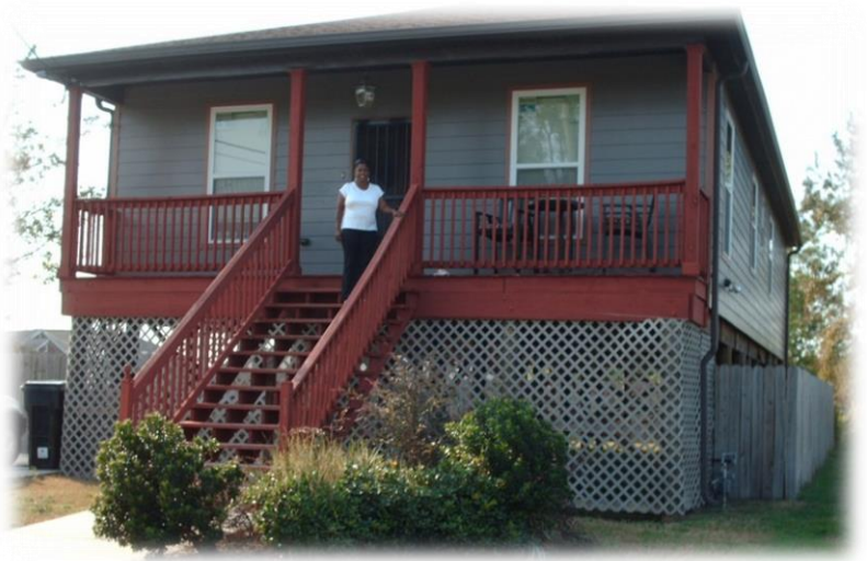
This home in New Orleans was elevated following a substantial-damage determination after Hurricane Katrina.
