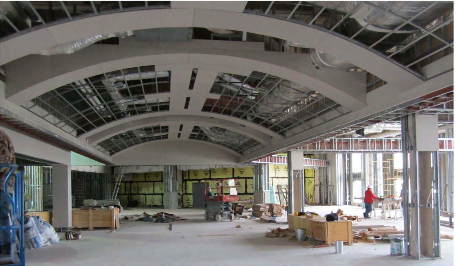
Installation of barrel ceiling at upper level Terminal Expansion
