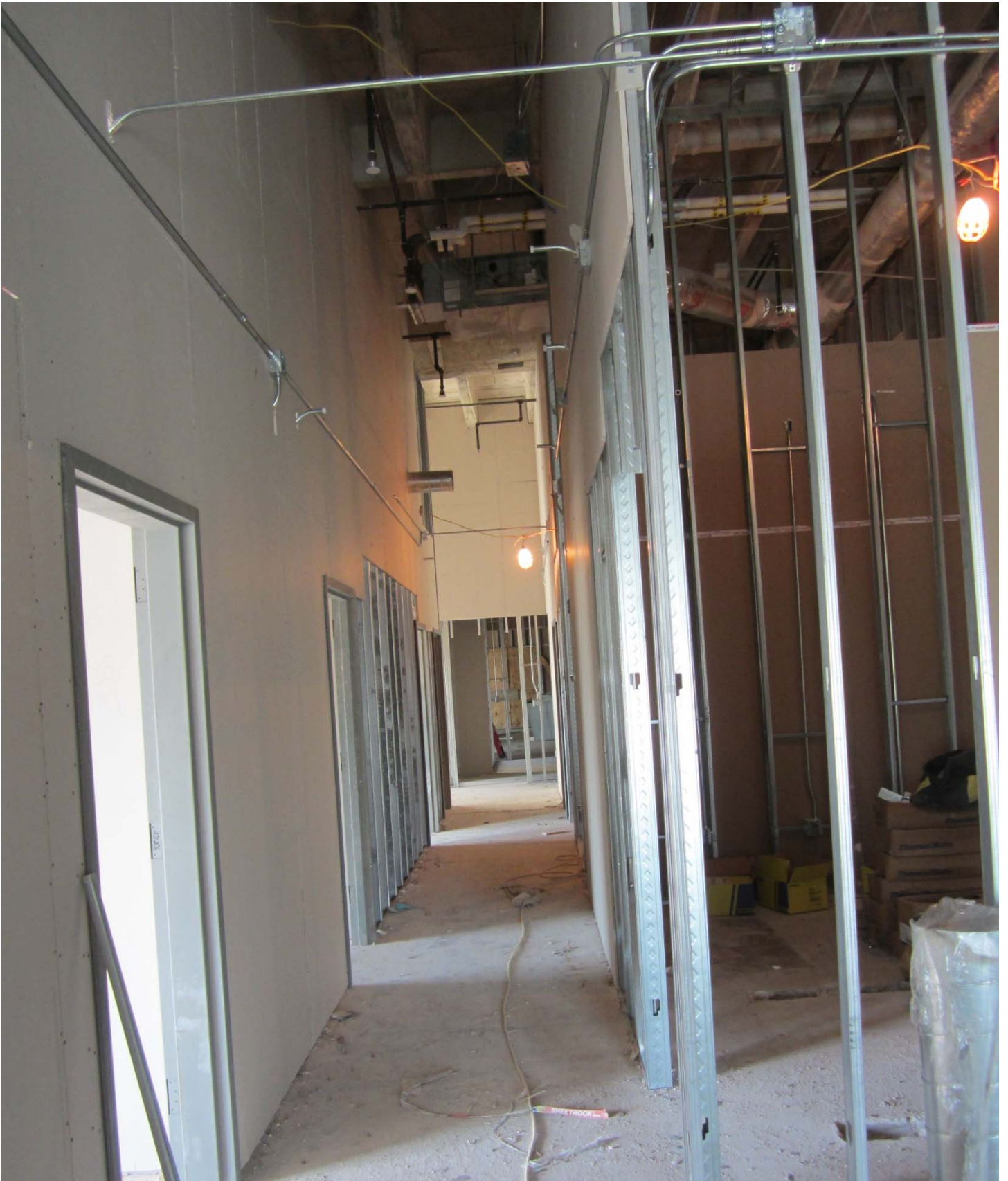
Wall framing and sheetrock installation for future TSA offices within the Terminal Expansion
