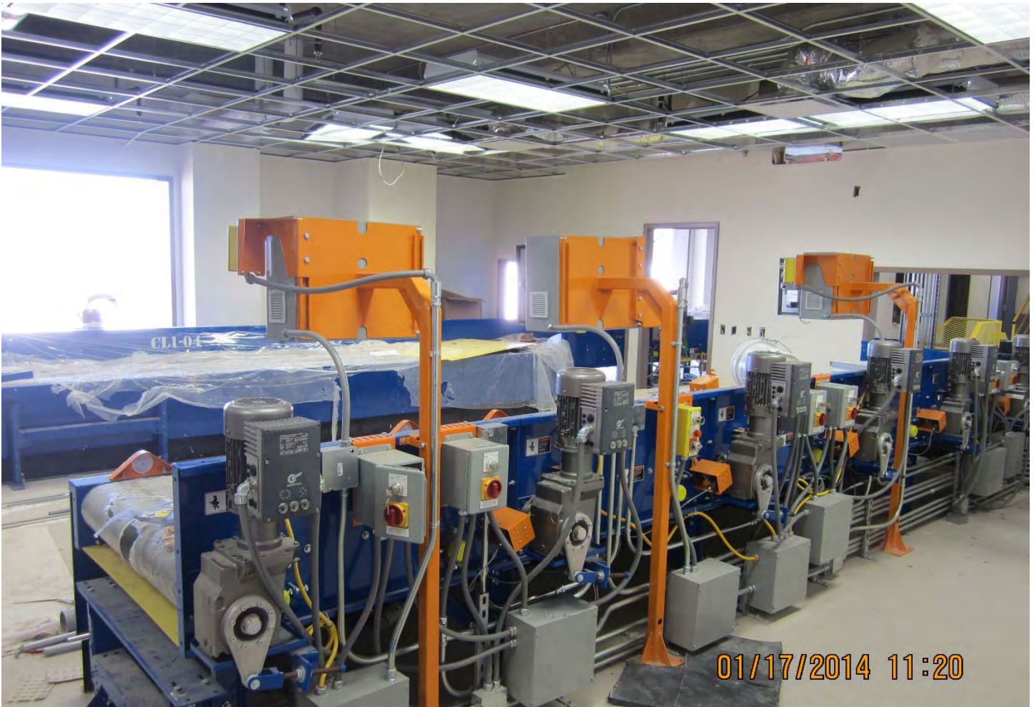
Continuation of TSA security equipment finish out at Baggage Handling Building
