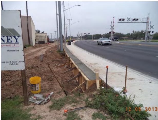
Screening Wall Foundation – Viewing North
