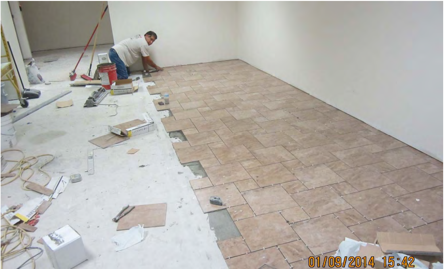
New tile installation in the General Aviation Federal Inspection Area Corridor
