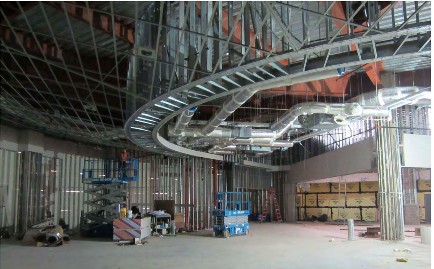
Radius Ceiling Framing at Rotunda within the upper level of the Terminal Expansion
