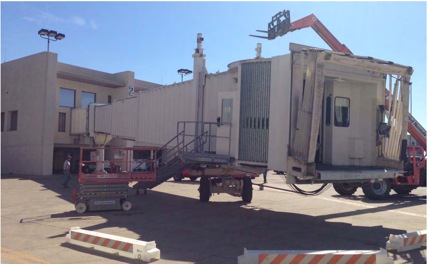
Commencement of Jet Bridge 2 refurbishments
