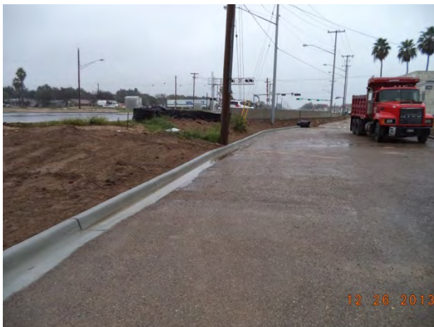
Curb & Gutter/Screening Wall – Viewing South
