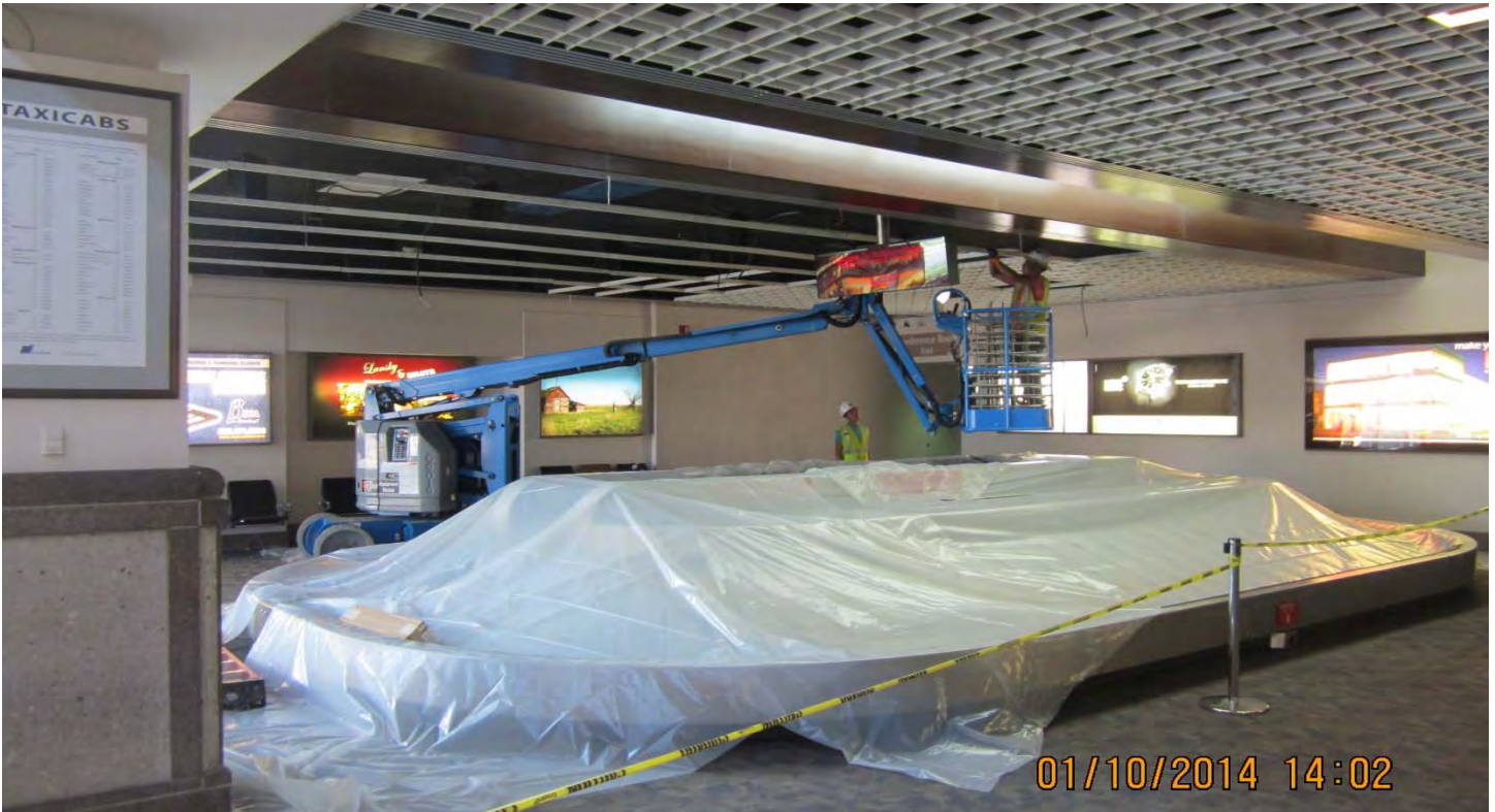
Ceiling reconstruction at baggage carousel within the existing Terminal
