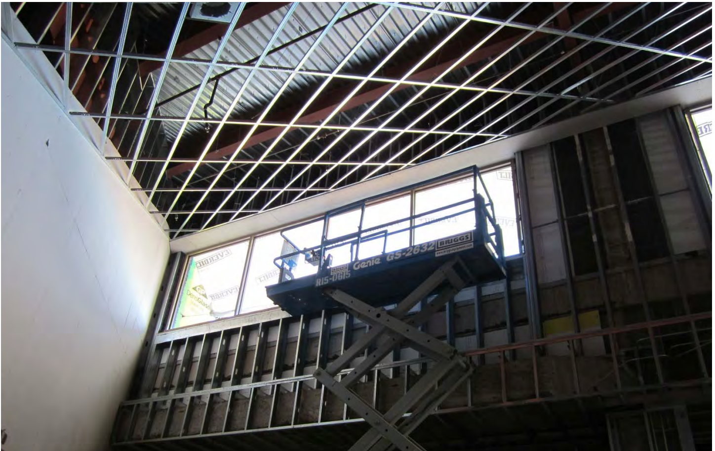
Installation of clerestory windows at upper level Terminal Expansion
