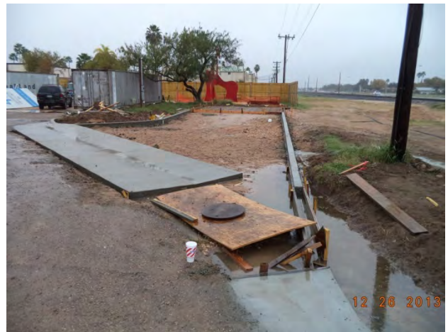
Dumpster Pad/Vehicle Queuing Area– Viewing North
