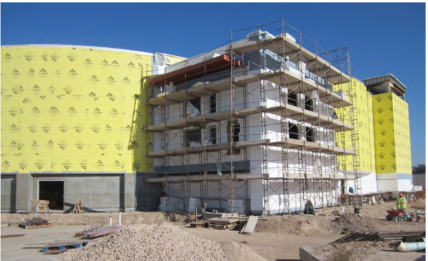
Insulation preparation for exterior EIFS at south east side of Terminal Expansion
