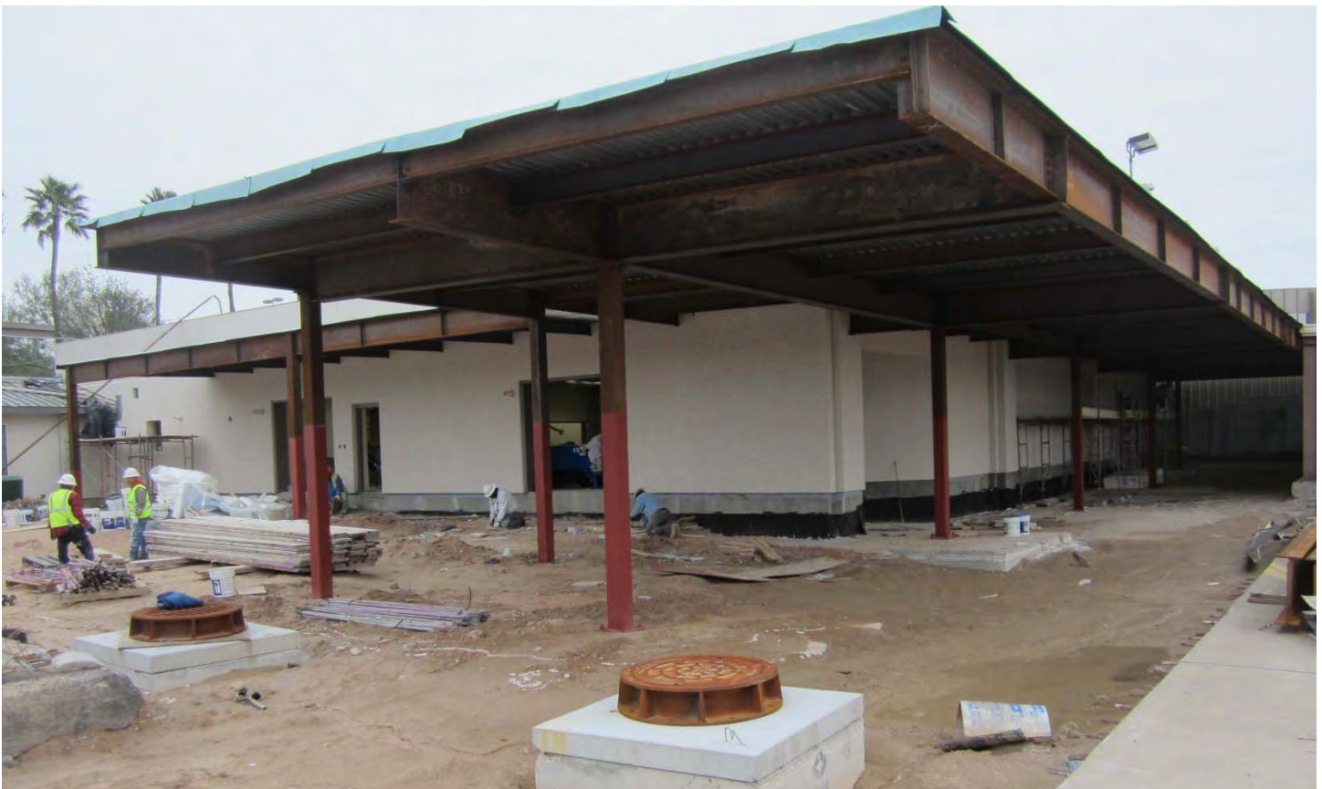
Finishing of exterior EIFS at the Baggage Handling Building
