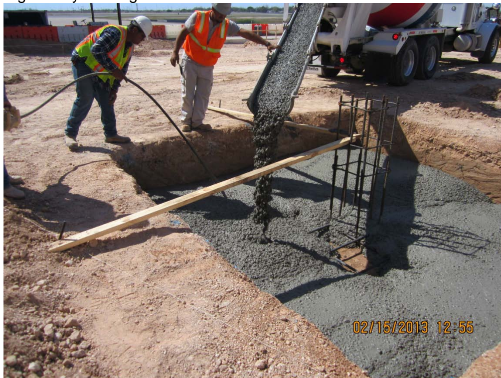
Baggage Handling Facility Footing Concrete
