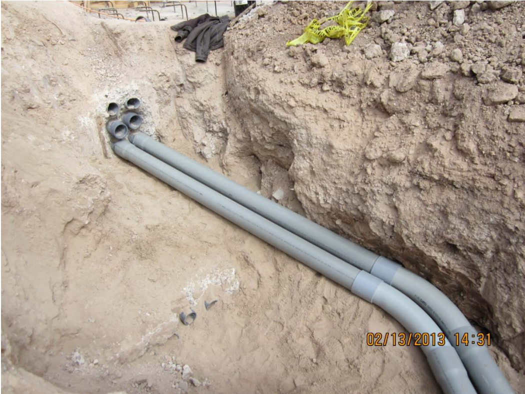
New Addition electrical Underslab Work
