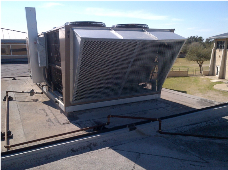
New Condenser Unit – Lark Community Center
