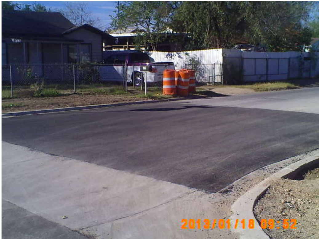
Drainage improvements complete. Curb reconstruction complete. Preparing for repairs to sidewalks and handicap ramps.
