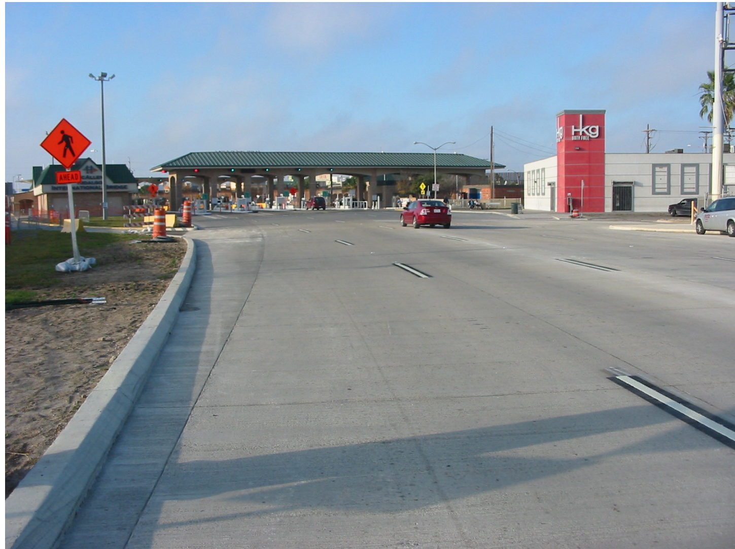
New concrete paving at Hidalgo Port of Entry looking southbound.
