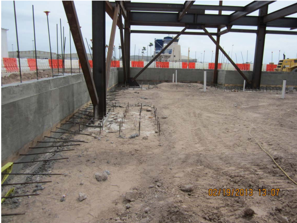
New Addition Perimeter Wall
