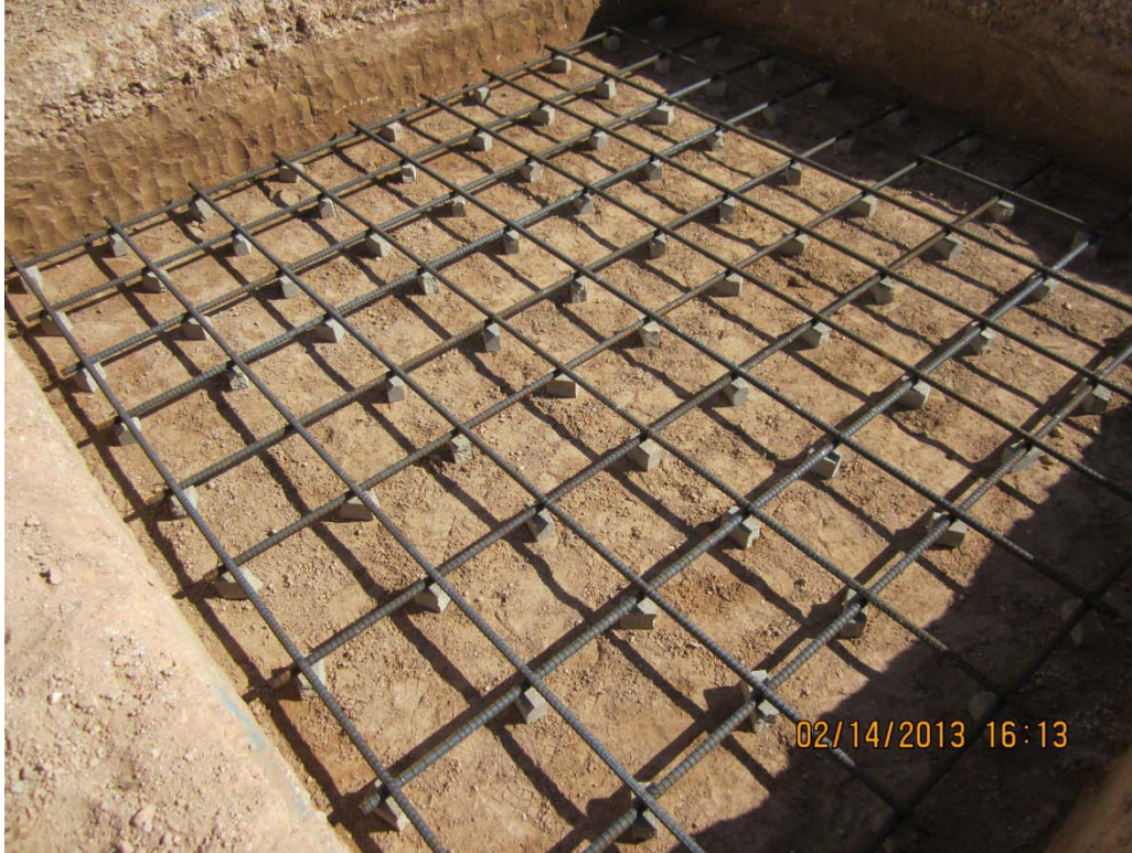
Baggage Handling Facility Footing Preparation
