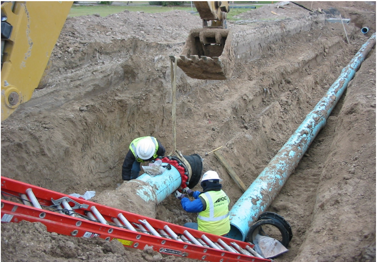
Utility crews adjusting 16-inch water main just north of Daffodil along the west side of Bentsen Road (looking north).
