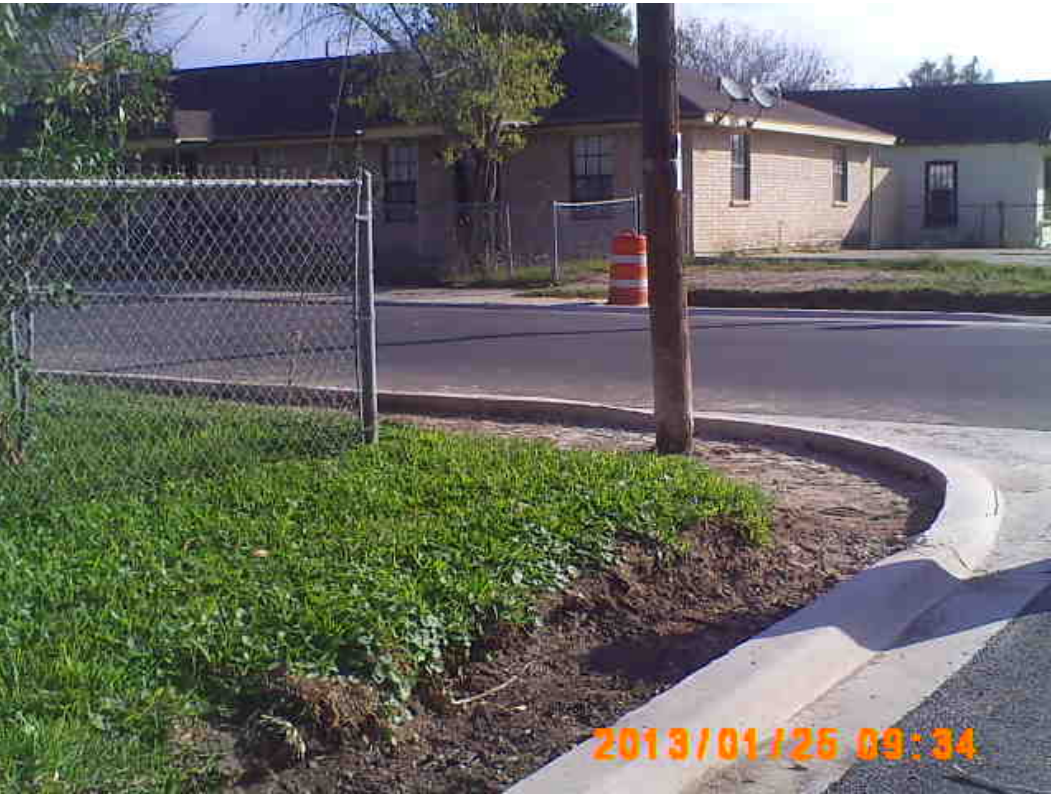
Improvements complete at intersection of Galveston and 22 nd . Six foot wide valley gutters constructed to allow flow to cross roadway and reduce ponding of stormwater at intersection.
