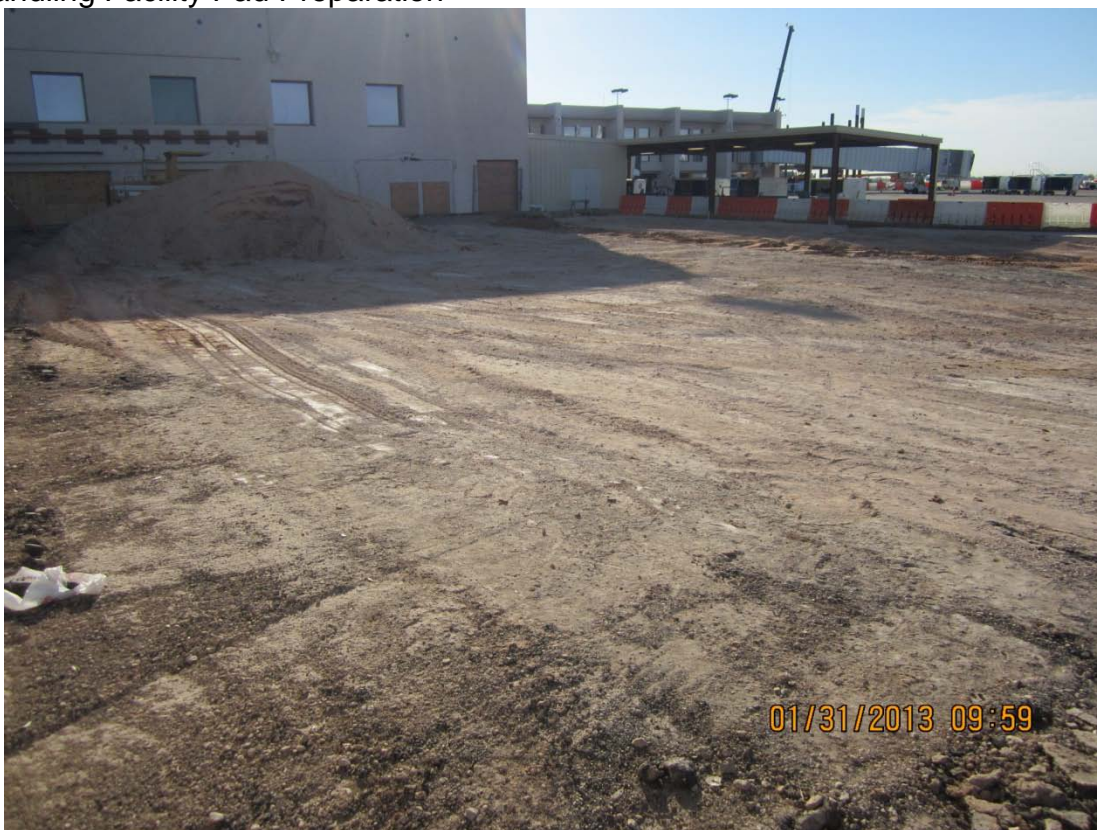
Baggage Handling Facility Pad Preparation
