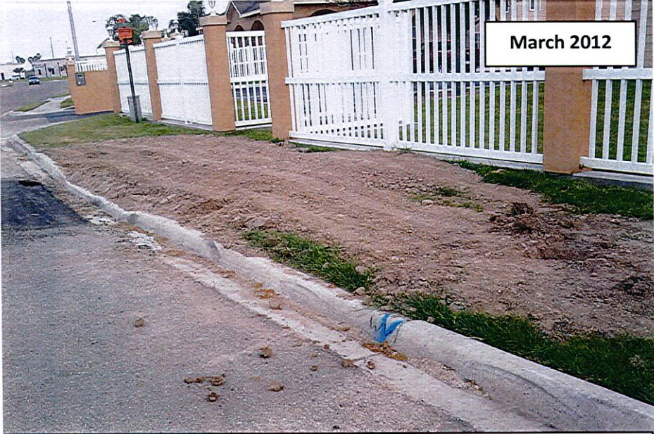
Redbud Avenue: North R.O.W. Repair Extents (Viewing NW)
