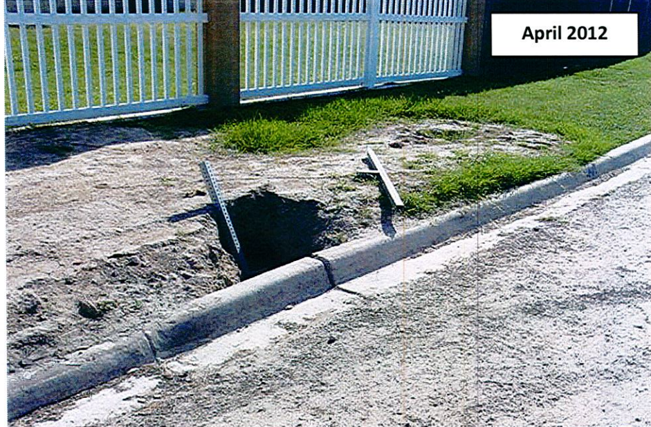
Redbud Avenue: Sinkhole at North R.O.W. (Viewing NE)
