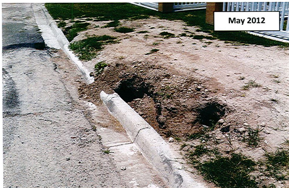
Redbud Avenue: Detail of Pavement Failure at North R.O.W.
