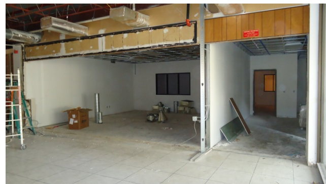
Removal of Tax Office Transaction Window
