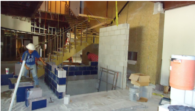
Elevator walls - construction
