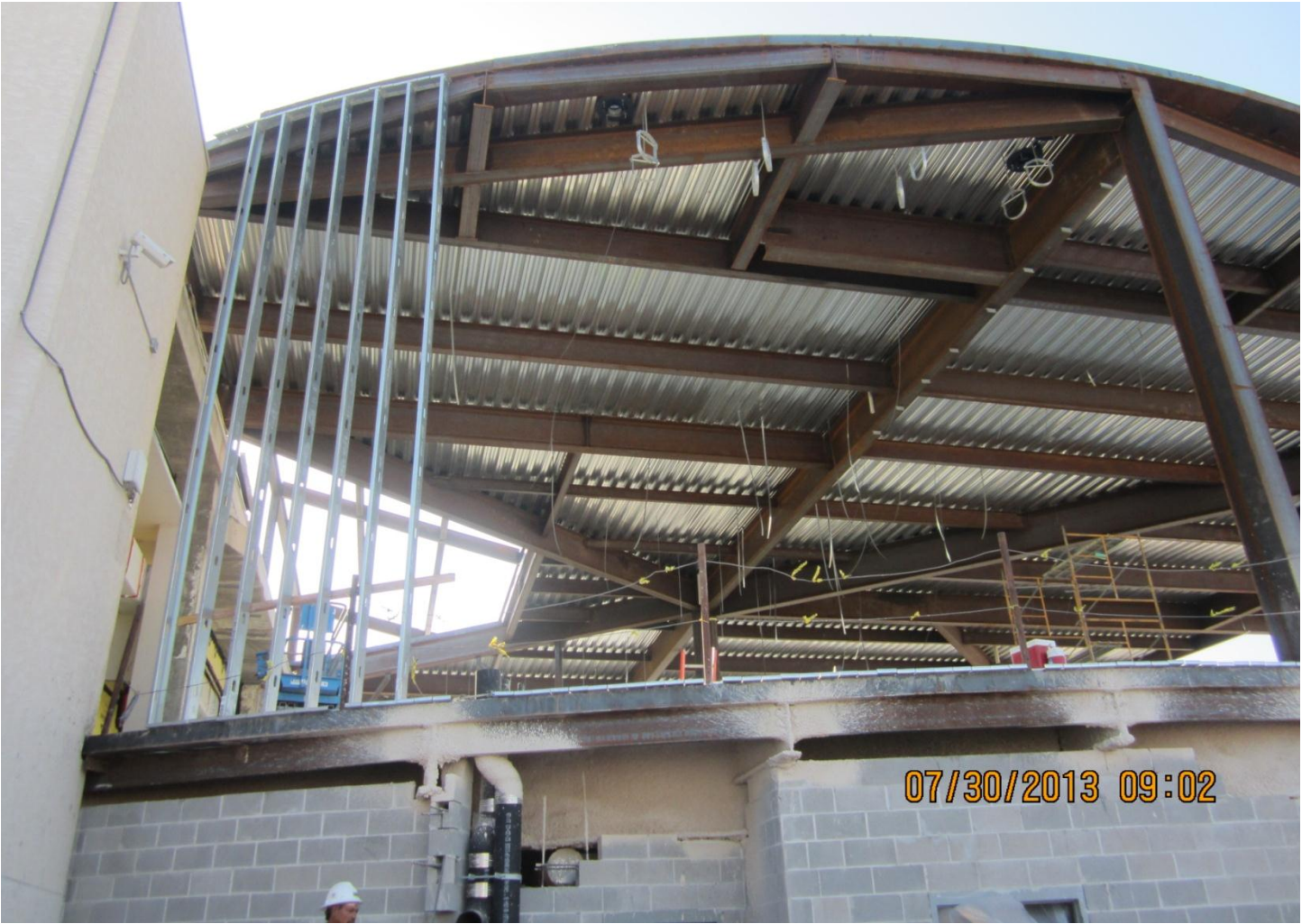
Metal stud framing of upper level of Terminal Expansion
