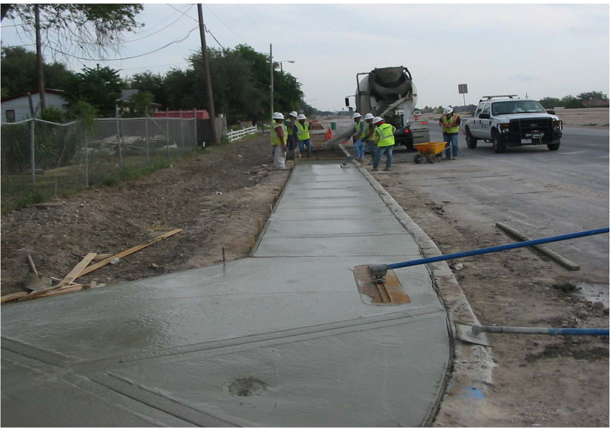
Sidewalk construction on the west side of Bentsen Road north of Daffodil.
