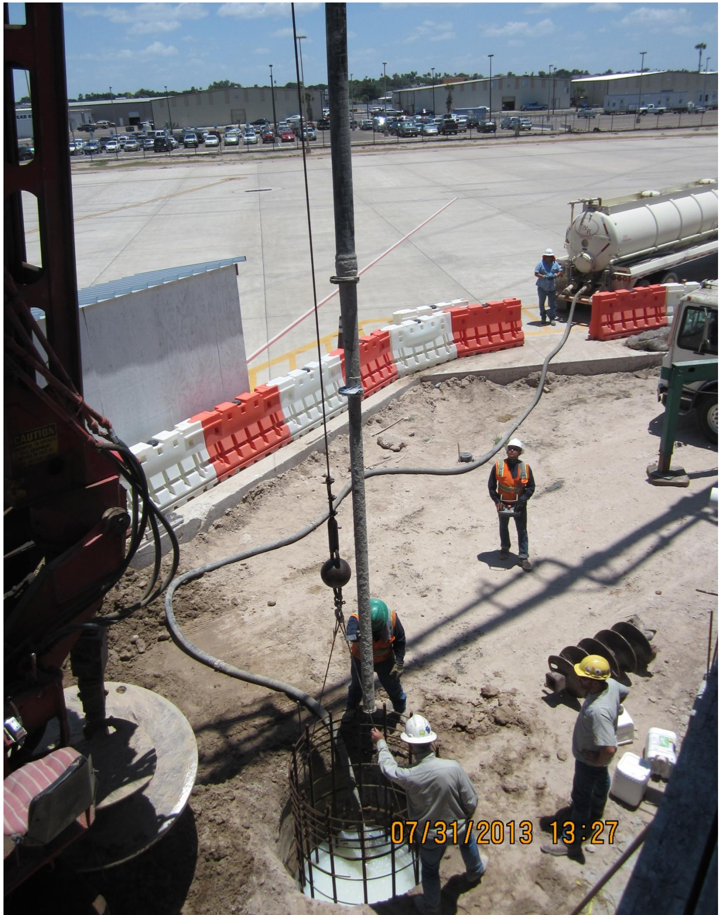
Foundation concrete pour for new jet bridge outside of Terminal Expansion
