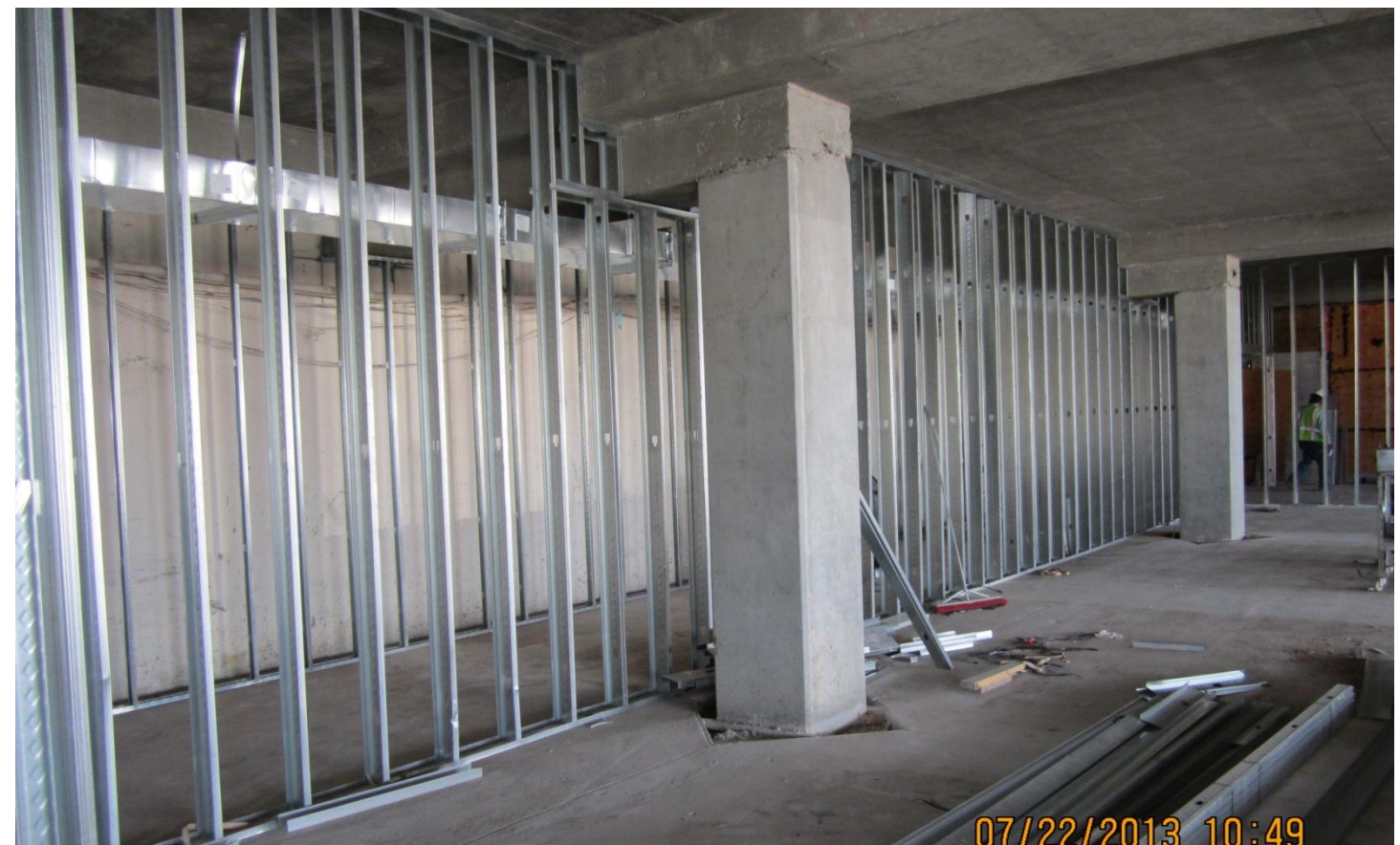
Metal stud framing within the Baggage Handling Building
