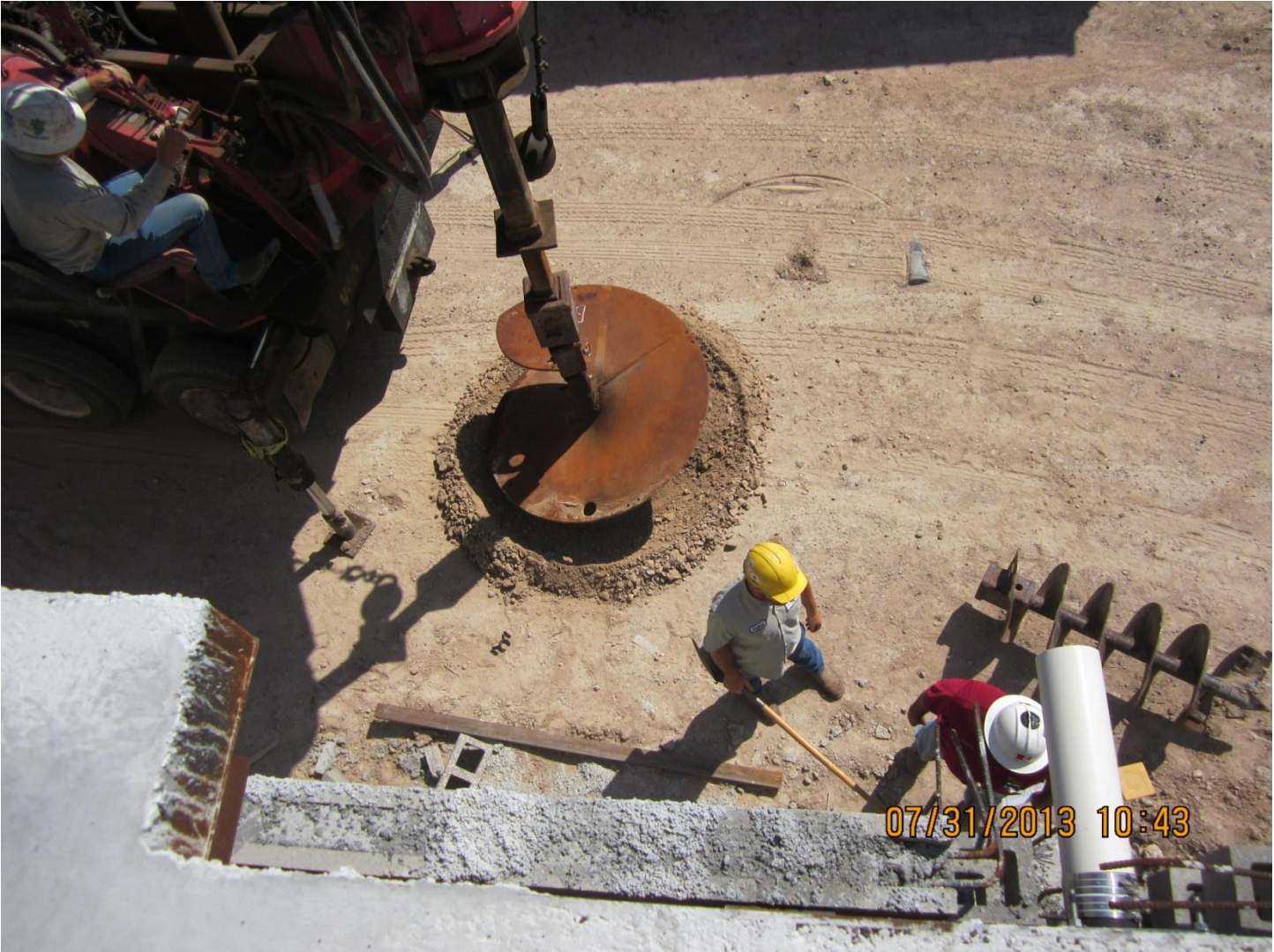
Drilling of foundation for new jet bridge outside of Terminal Expansion
