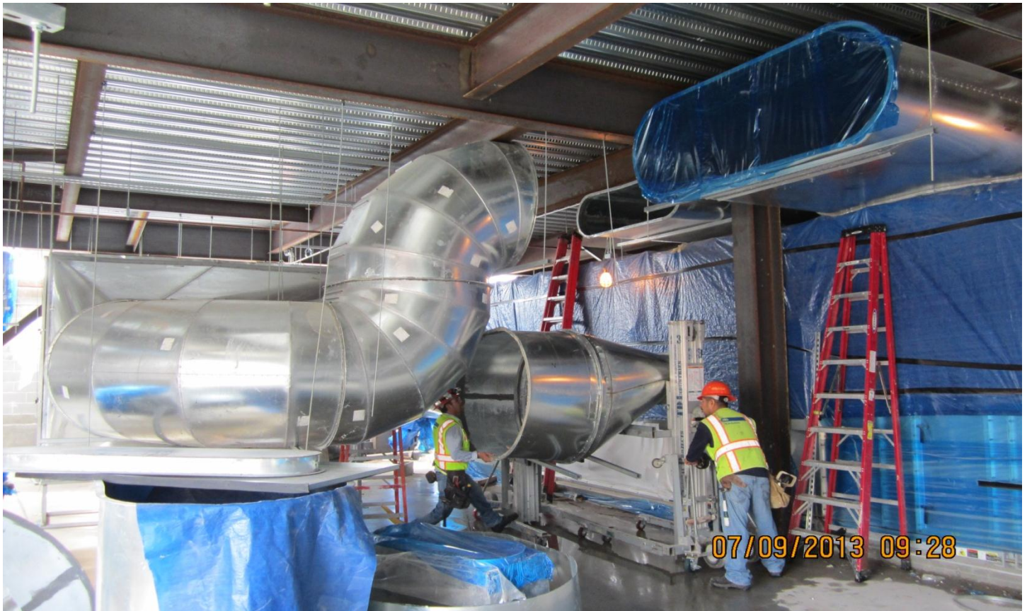
Installation of HVAC ductwork on lower level mechanical room of the Terminal Expansion
