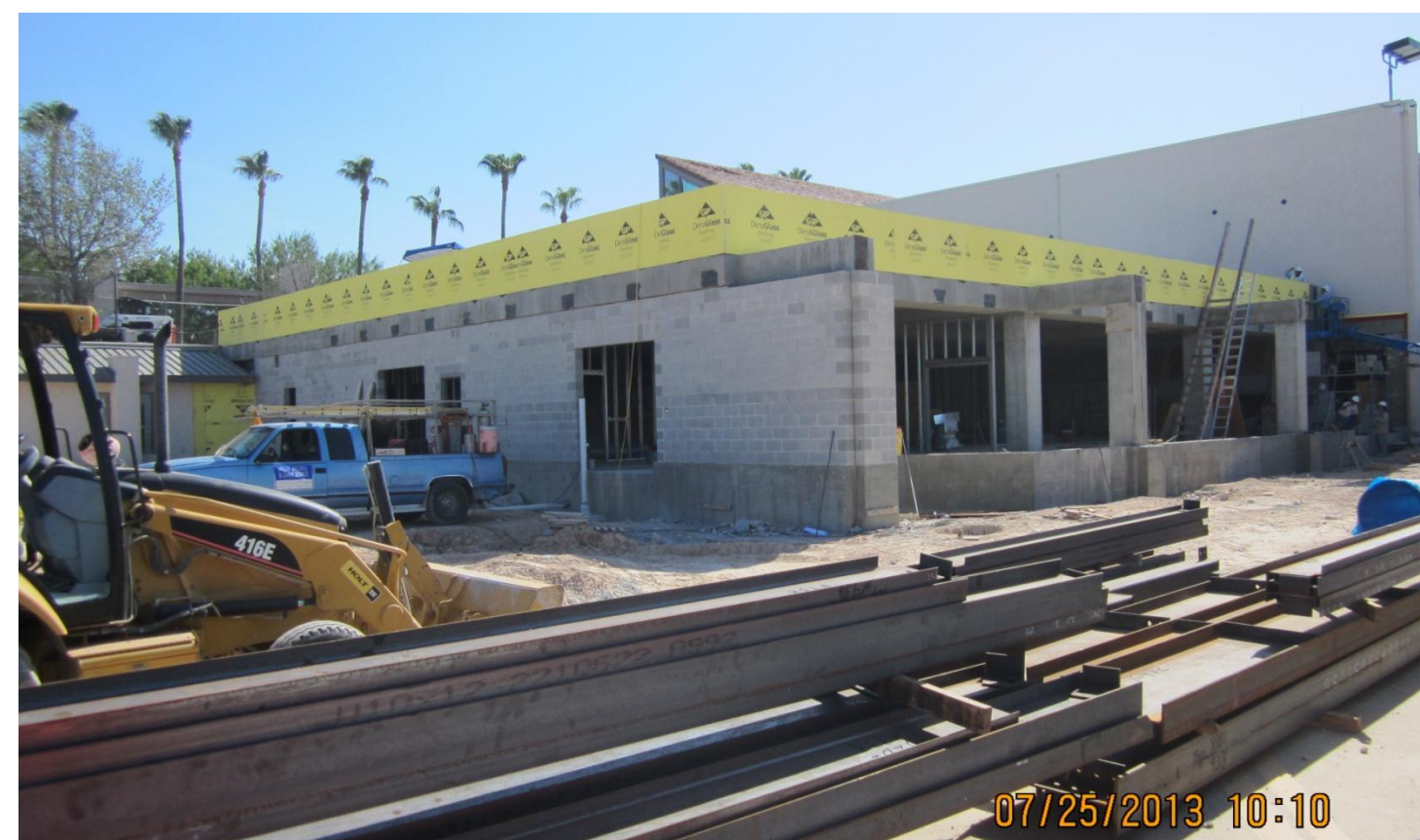
Covering of parapet wall at Baggage Handling Building
