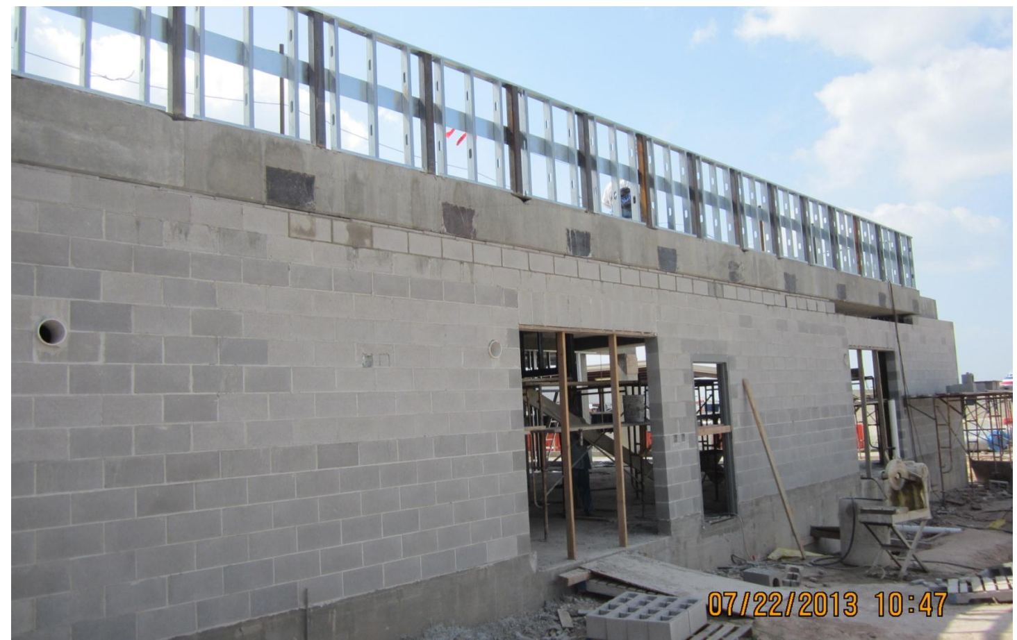
Metal stud framing within the Baggage Handling Building
