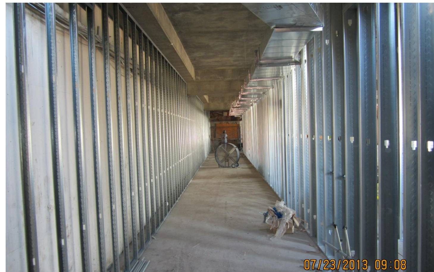
Metal stud framing and HVAC ductwork within GA FIS walkway at the Baggage Handling Building
