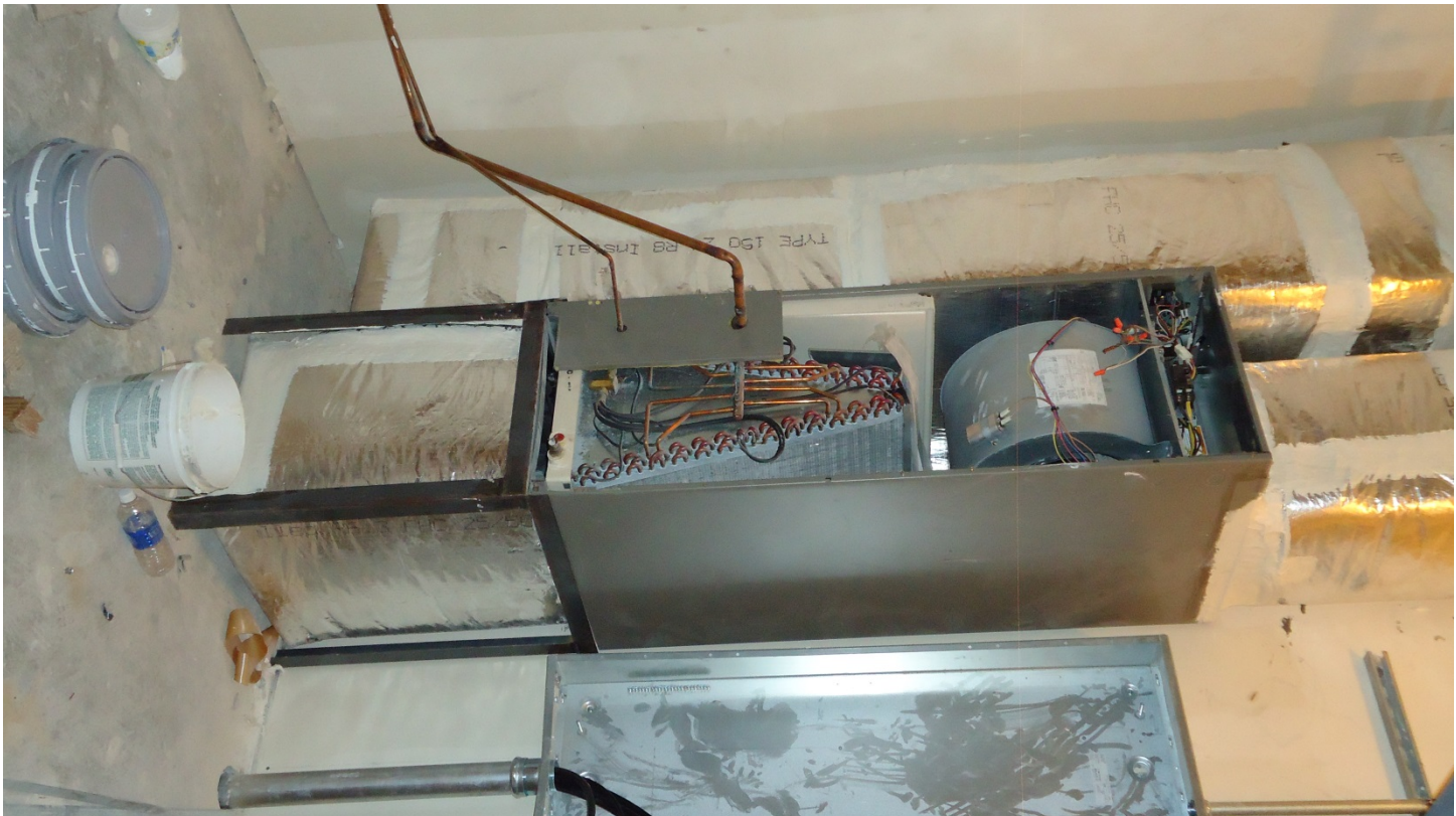
Typical HVAC (air handling equipment) throughout several areas of the building
