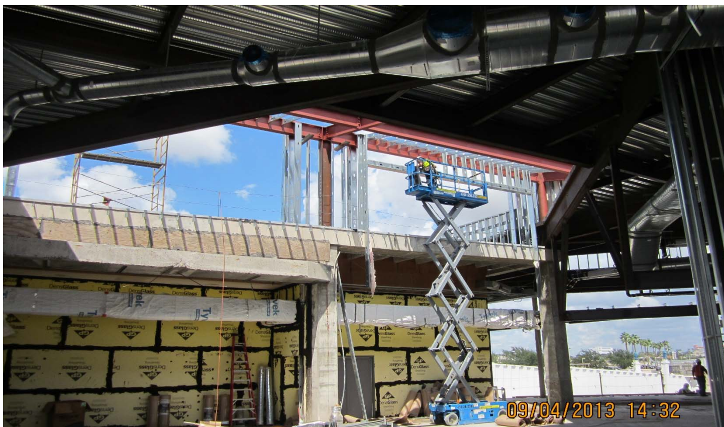
Metal stud framing at upper level of Terminal Expansion
