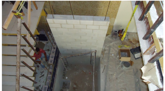
View into elevator shaft from above
