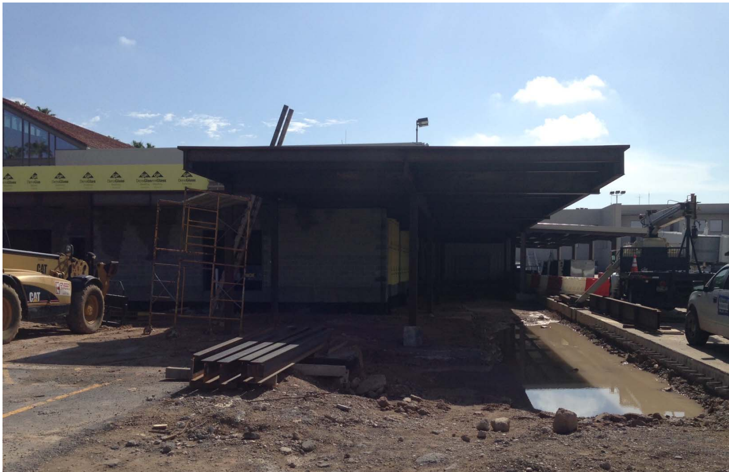
Canopy of Baggage Handling Building from west end view
