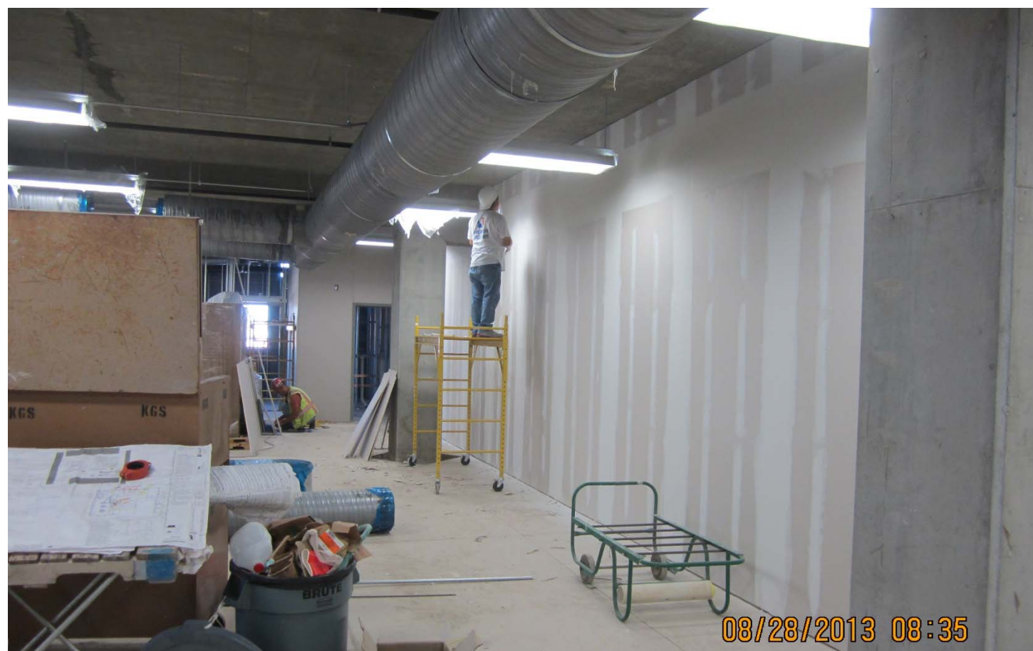
Joint sealing of interior walls at the Baggage Handling Building
