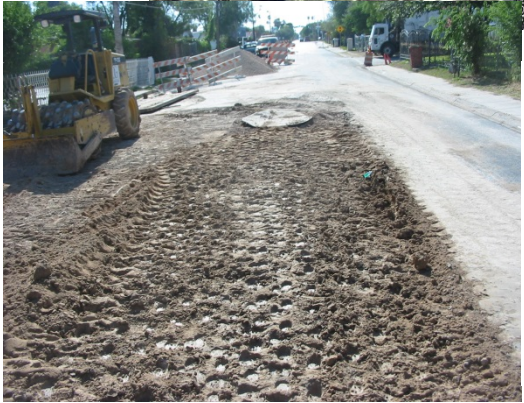
Top: Map of contractor's progress. Left: Compaction of subgrade along Hackberry Ave. Right: Installation of storm sewer.
