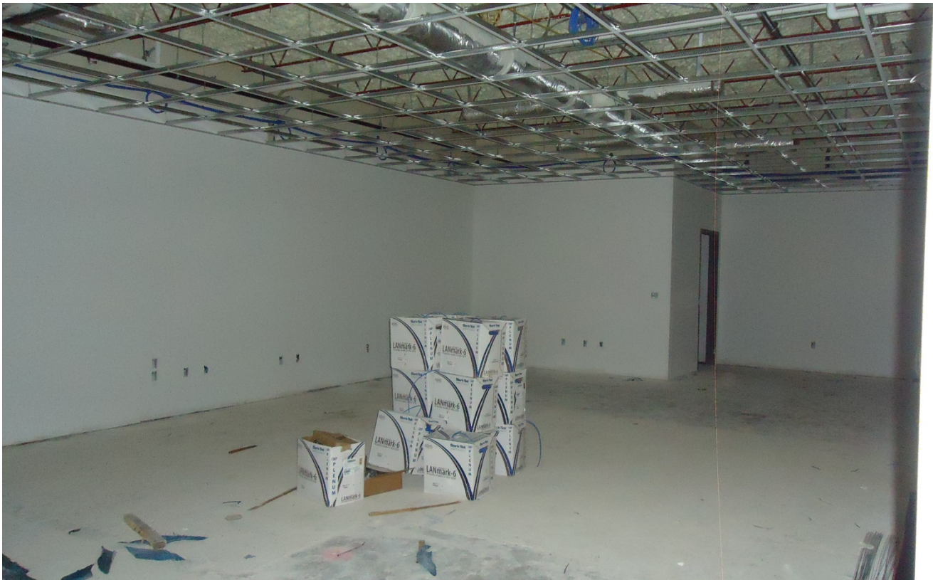
Placement of ceiling grid is in over most spaces now. Data cabling continues.
