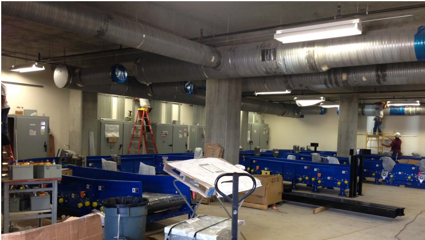
Installation of the baggage handling equipment at the Baggage Handling Building
