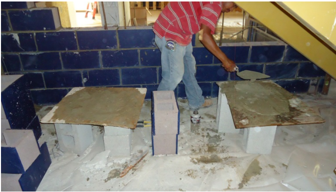
Glazed block placement at elevator shaft
