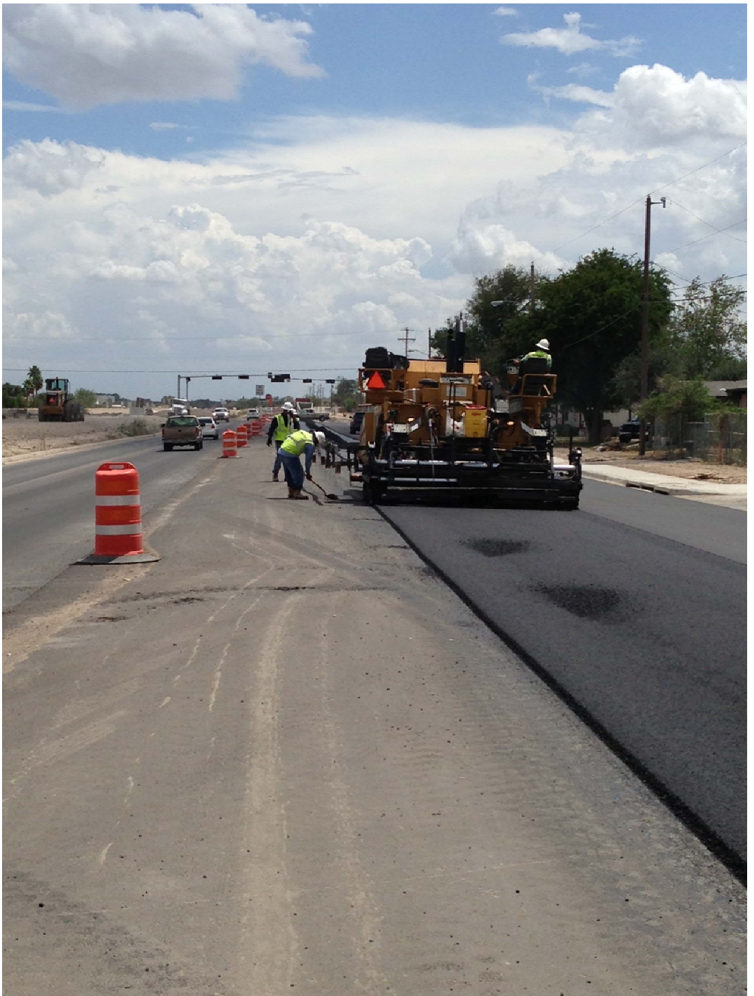
Final pavement lift on future southbound lanes just north of Daffodil.
