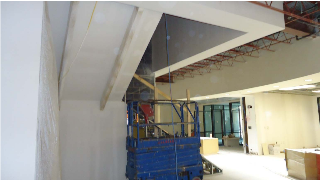
Photo taken facing NE from under stair; new conference area in background.
