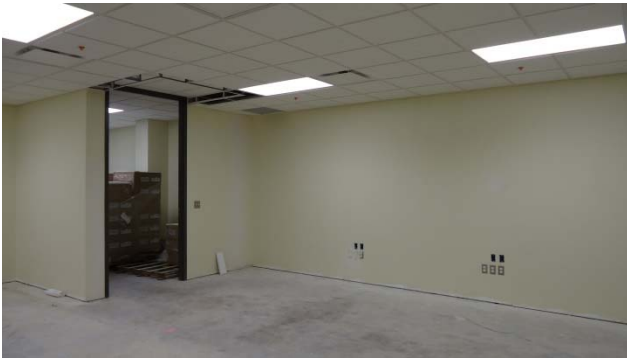
Painting and ceiling tile – room C104
