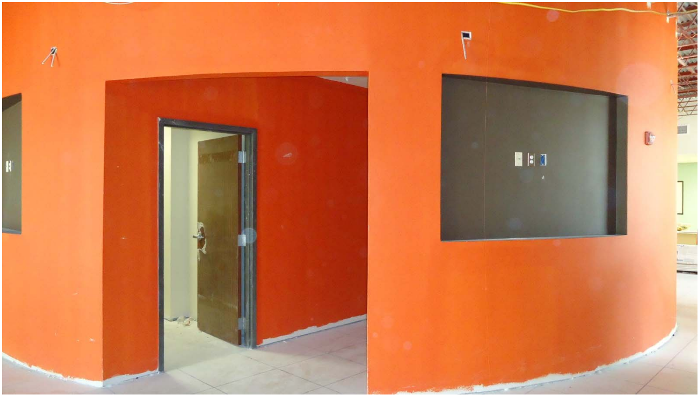
The central core; door to elevator machine room; recessed areas for monitor installations
