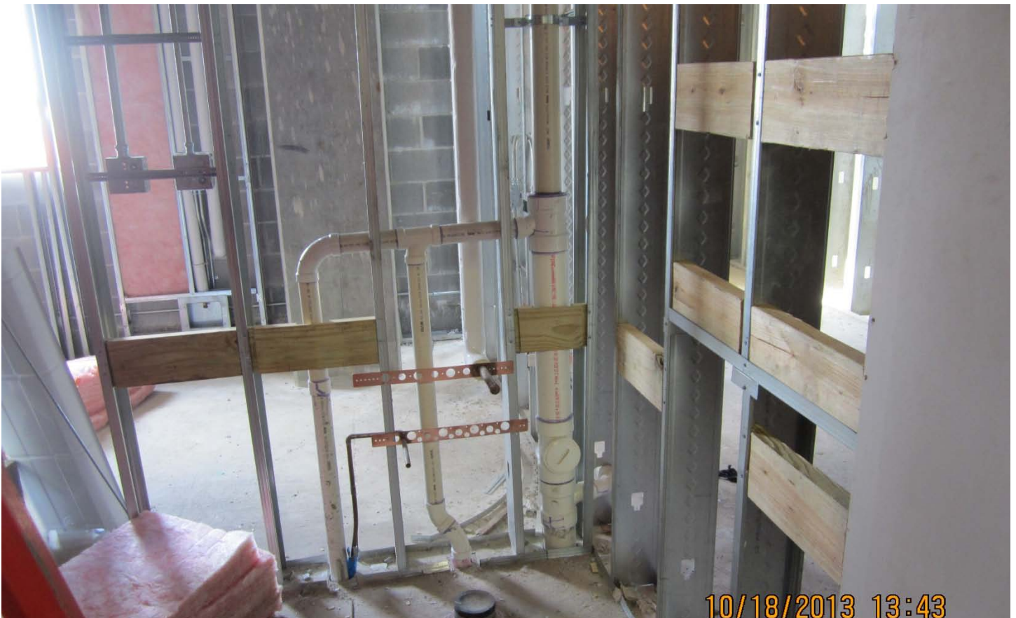
Plumbing work within the Baggage Handling Building
