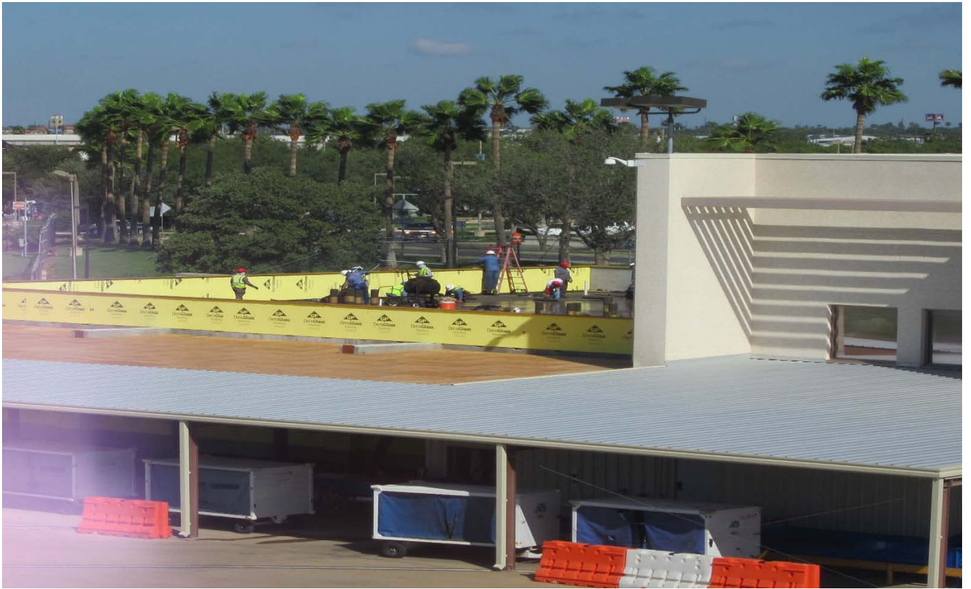
Roof work at the Baggage Handling Building
