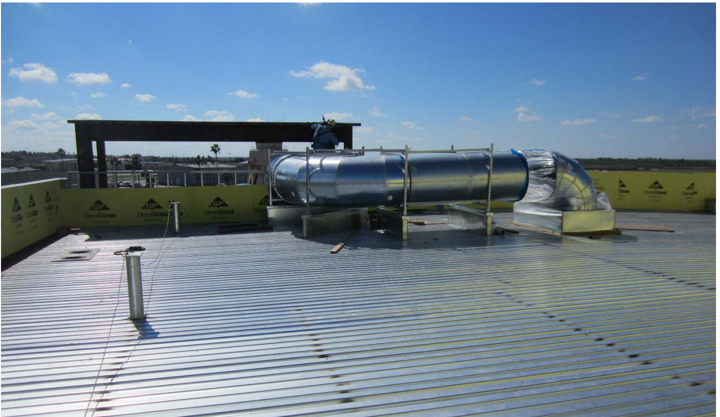
HVAC ductwork on roof of upper level at Terminal Expansion
