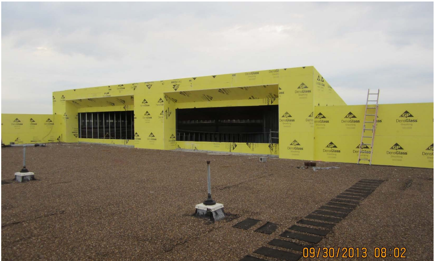
Installed sheathing for clerestory window at roof level of Terminal Expansion
