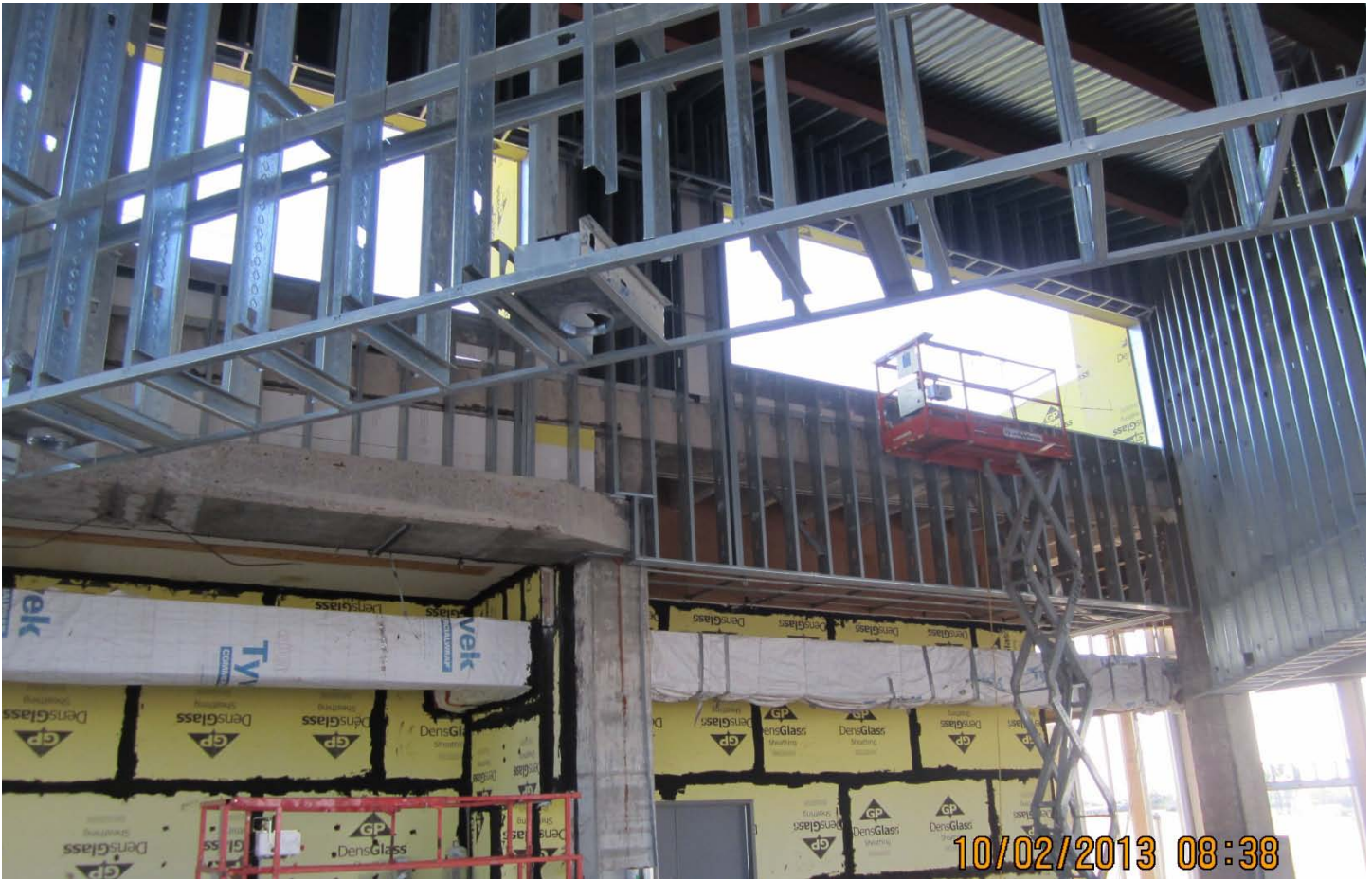
Interior metal stud framing at upper level of Terminal Expansion
