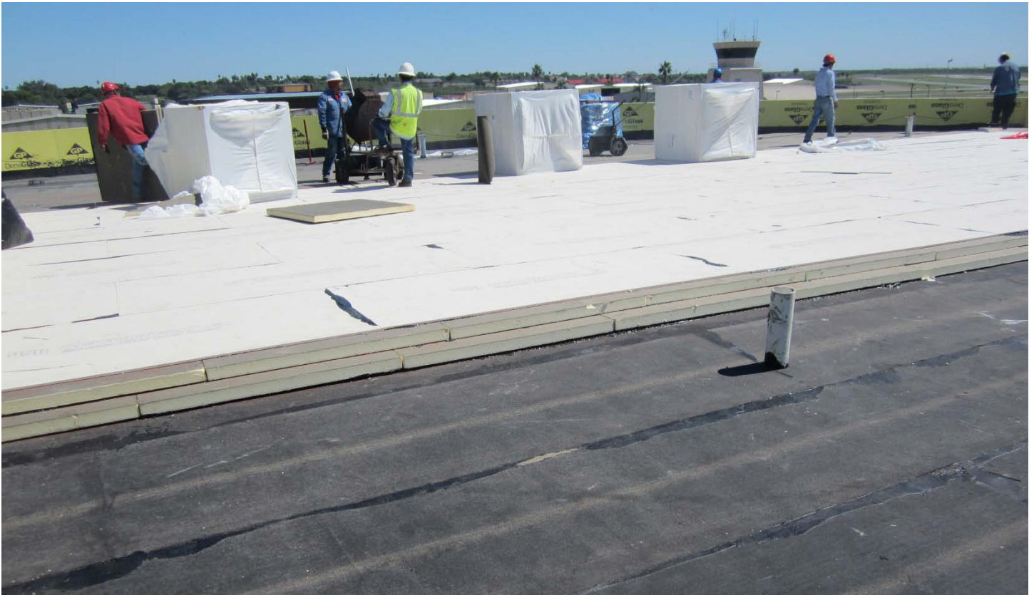
Installation of insulated tapered roofing system at Terminal Expansion
