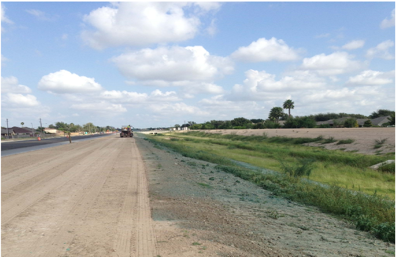
Final seeding of existing Mission/McAllen Lateral Ditch.
