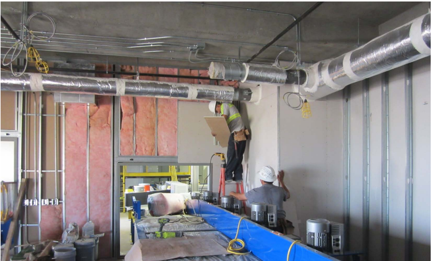
Installation of ductwork above conveyors at the Baggage Handling Building
