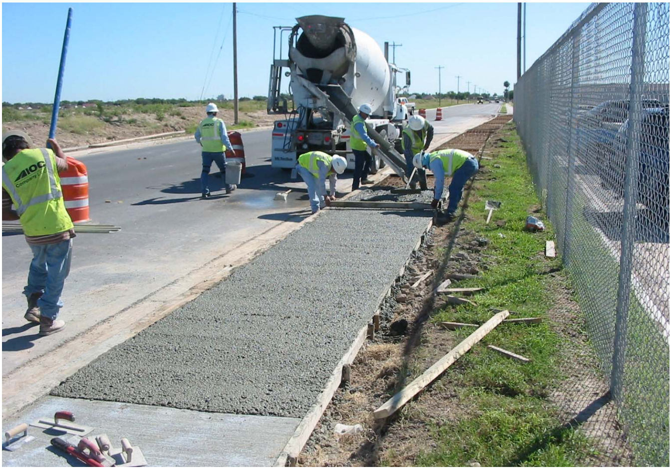
Sidewalk construction along the south side of Vine extension.
