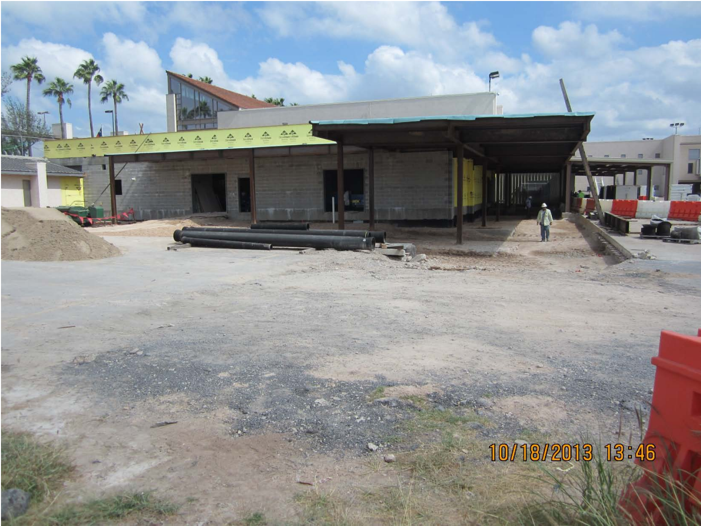
Canopy of Baggage Handling Building from west end view
