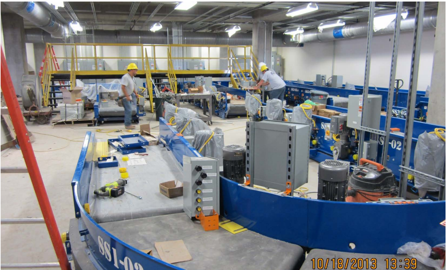
Installation of baggage handling equipment at the Baggage Handling Building
