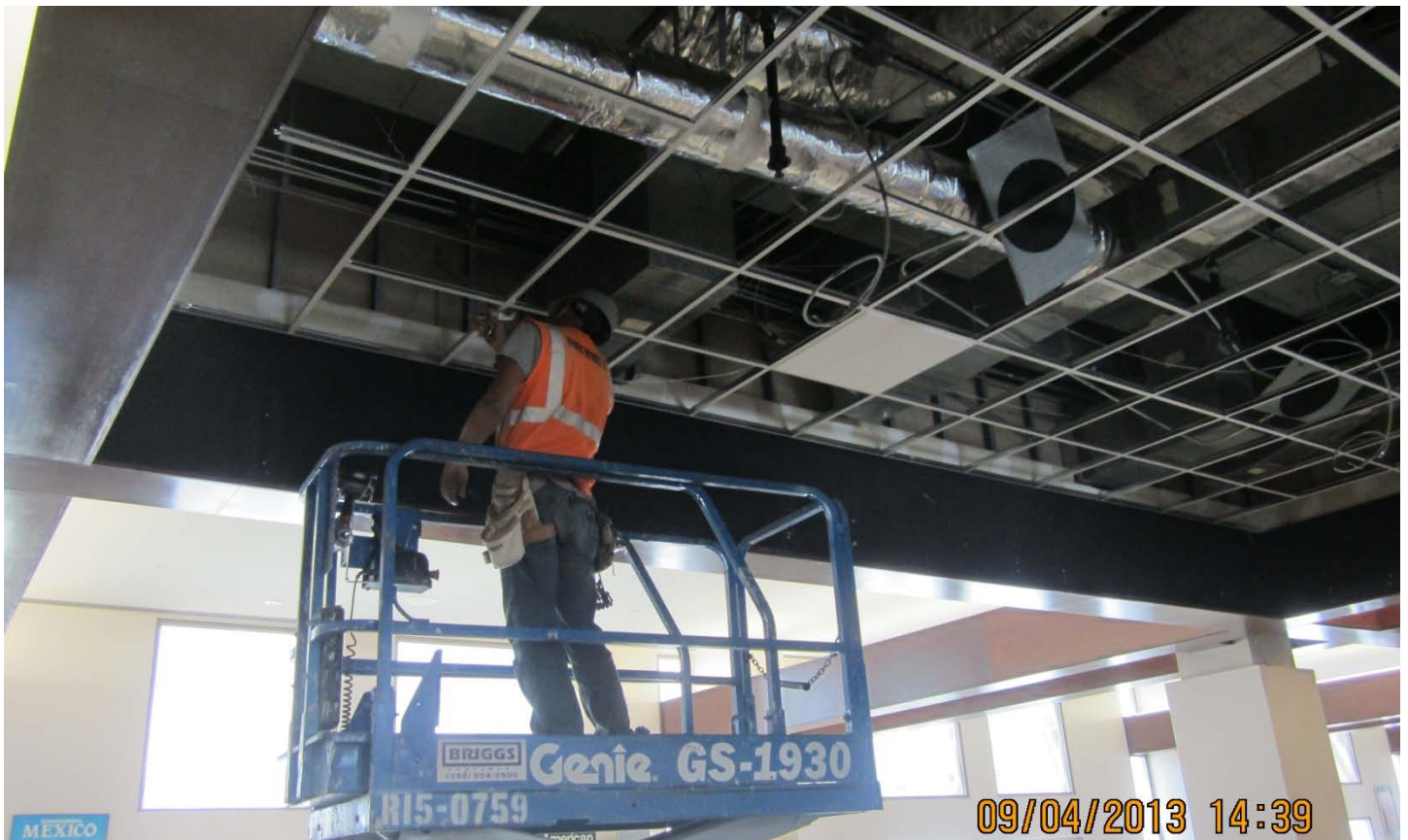
Ceiling work within the Terminal Expansion
