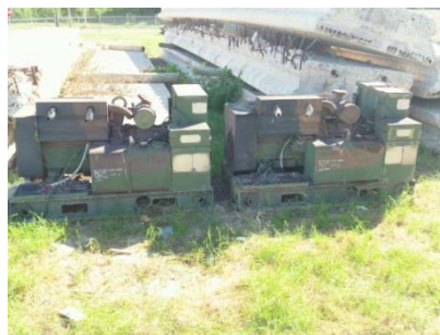
Diesel Engine Generators
