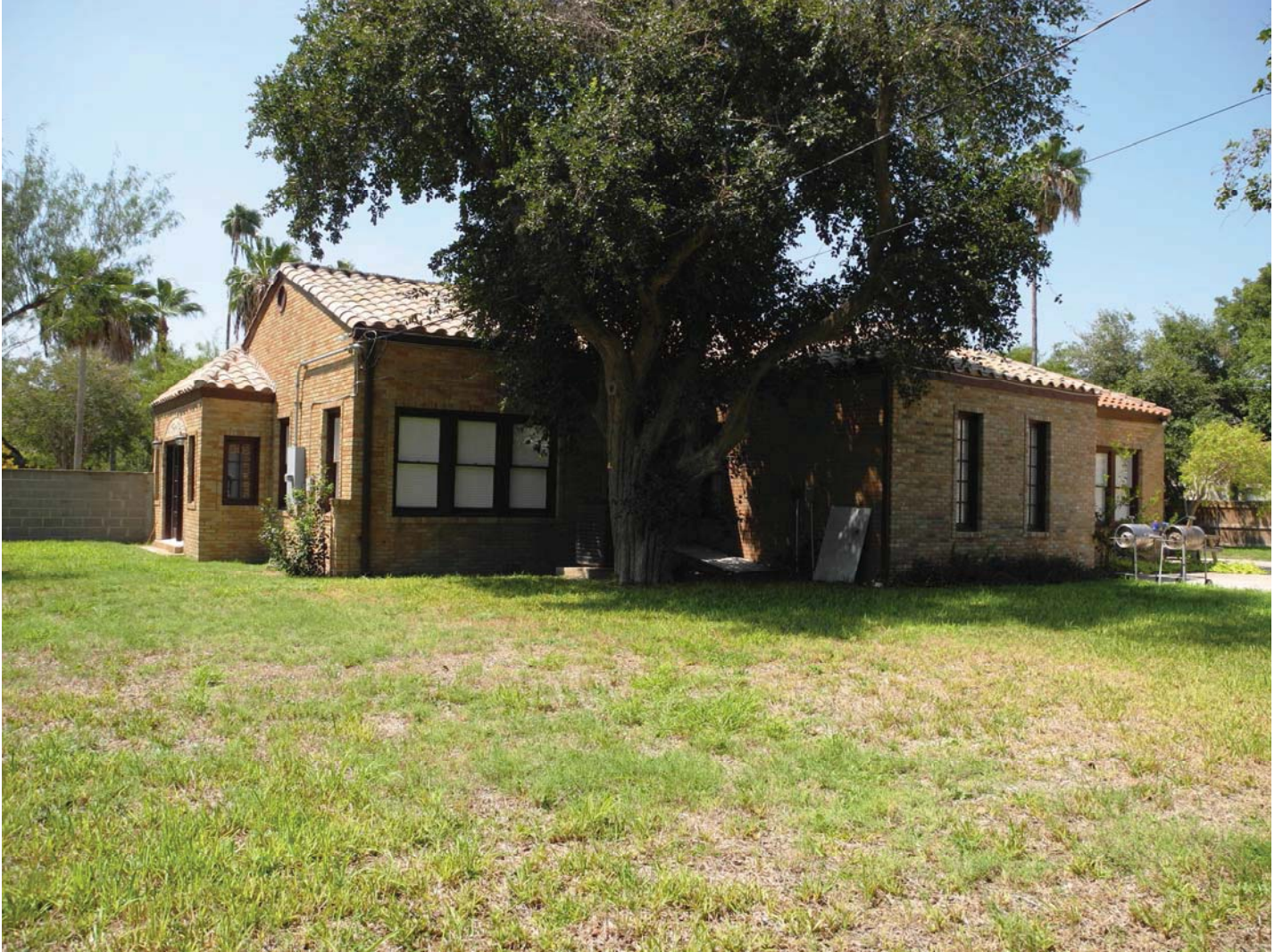
Photograph 5: East façade showing addition and original bedroom, Camera facing NW.
