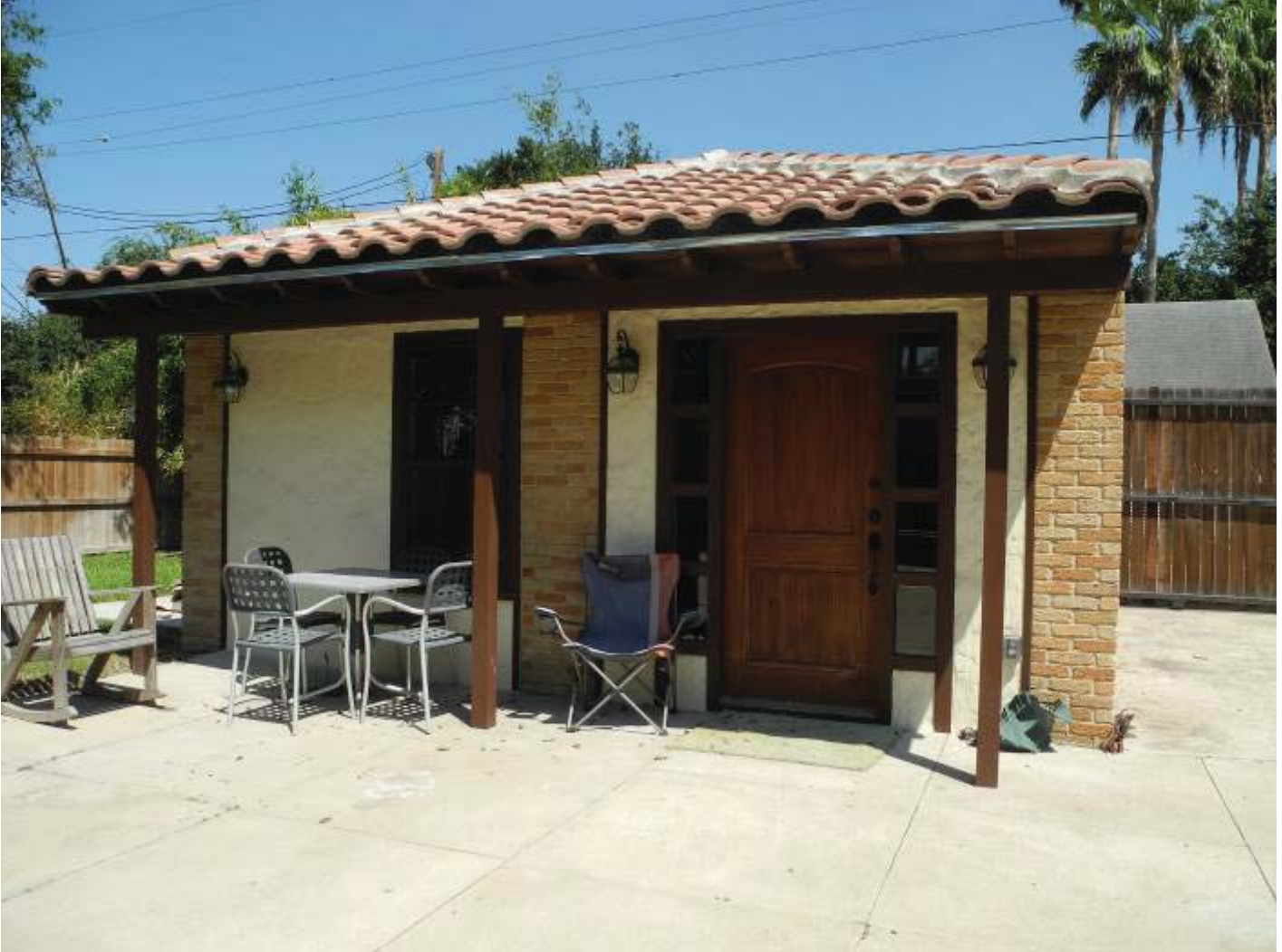
Photograph 7: Noncontributing garage, camera facing east.
