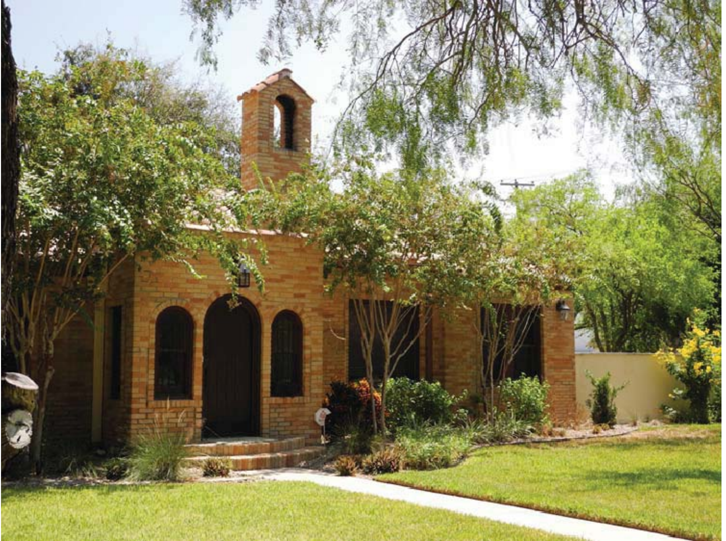
Photograph 2: Cluster of Spanish Colonial Revival features at entrance, camera facing SE
